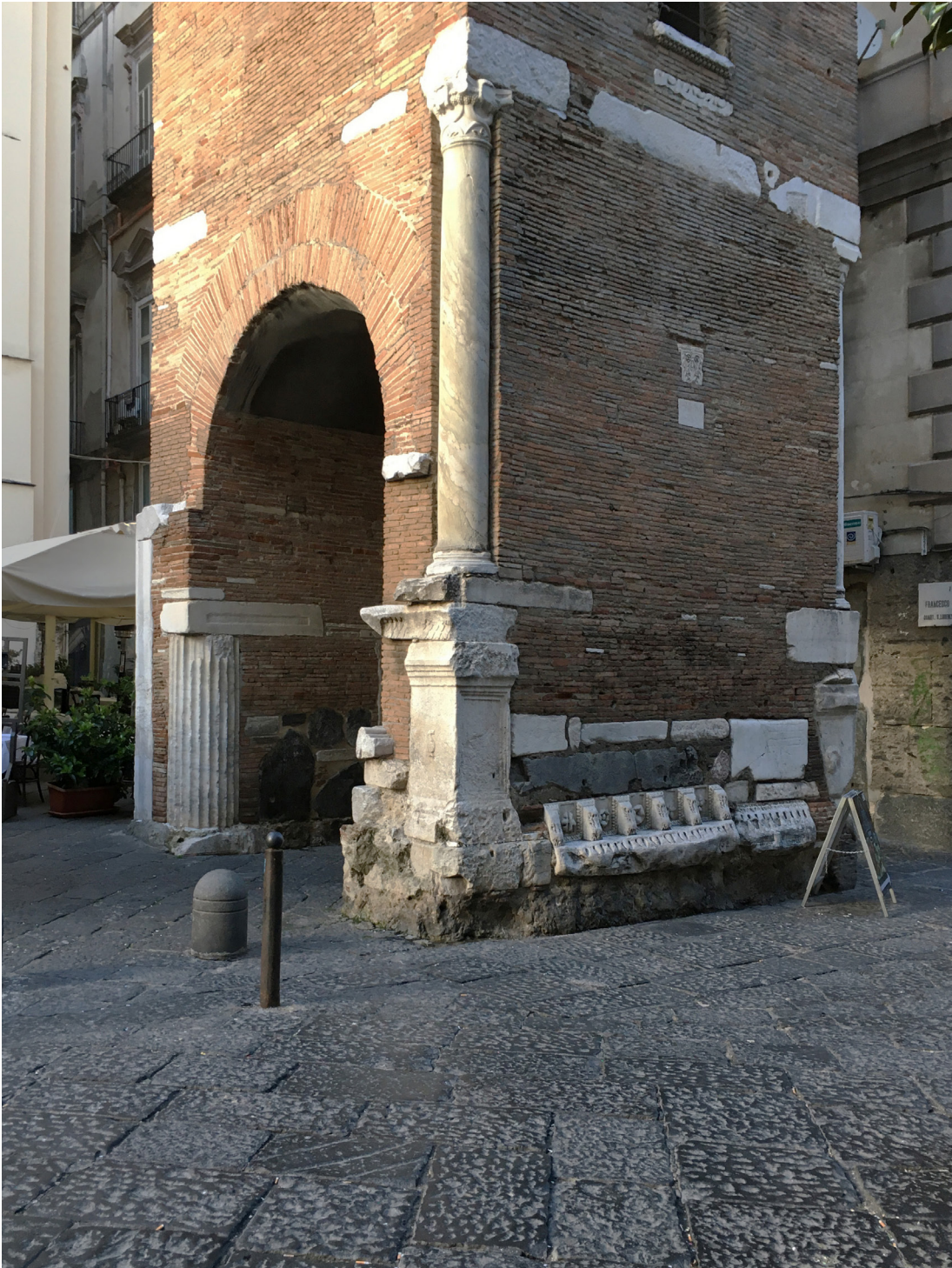
Fig. 1: Incorporation of marble fragments of antiquity in the medieval bell-tower (probably dated from the ninth or tenth century) of Santa Maria Maggiore della Pietrasanta, Naples. Photo: author.
