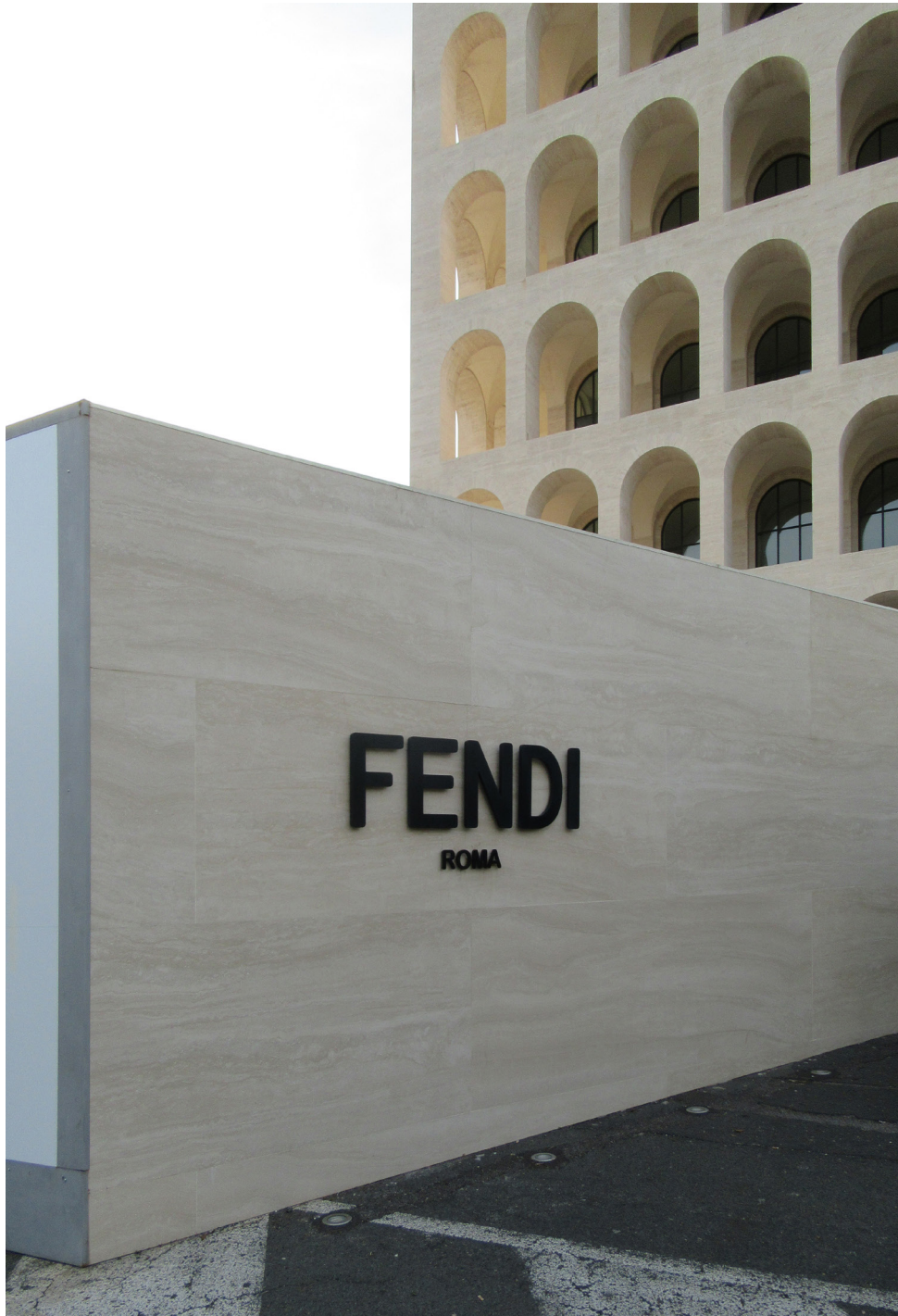
Fig. 7: Inscribed by a quotation from Mussolini's declaration of war on Ethiopia: The Palazzo della Civiltà Italiana, completed in 1940 in the EUR district in Rome, serves as the headquarters of the Italian fashion house Fendi since 2015 and appears as a stylish setting in advertising videos. Photo: Stephan Trüby.
