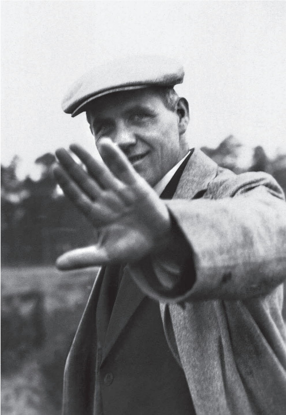
Fig. 1: Hannes Meyer at the site of the Federal School of the General Trade Unions (ADGB) in Bernau near Berlin (1928). Photo: Erich Consemüller(?), Stephan Consemüller, Stiftung Bauhaus Dessau.
