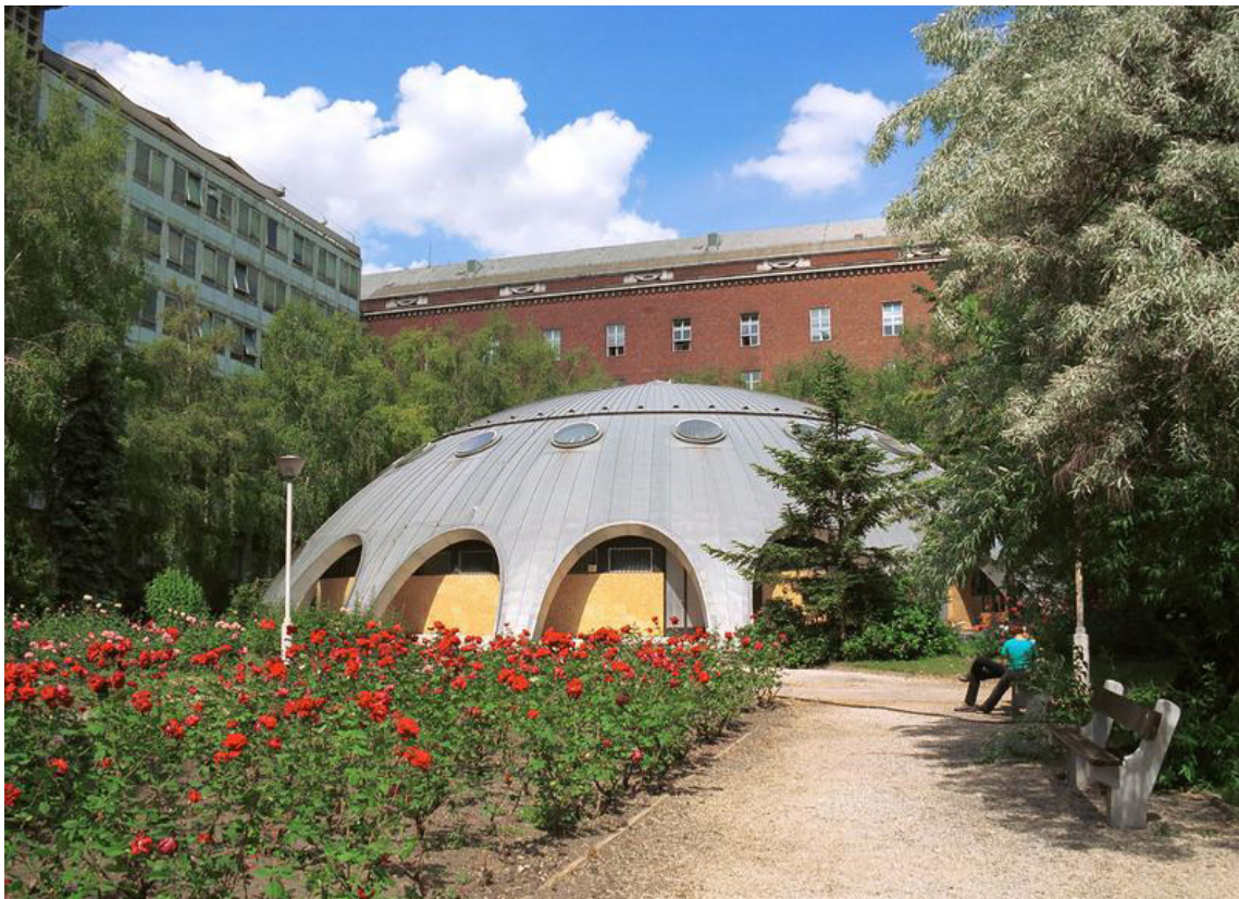
Fig. 1: Façade of Building R, Budapest University of Technology and Economics (detail). Plan: Plan Archive of Budapest Technology and Economics.
