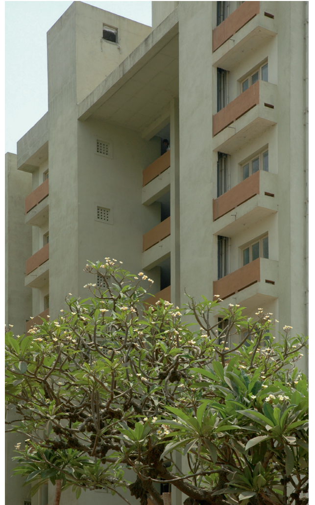
Sangharsh Nagar, appartementen- blok, vlak na voltooiing Sangharsh Nagar apartment block, just after completion
