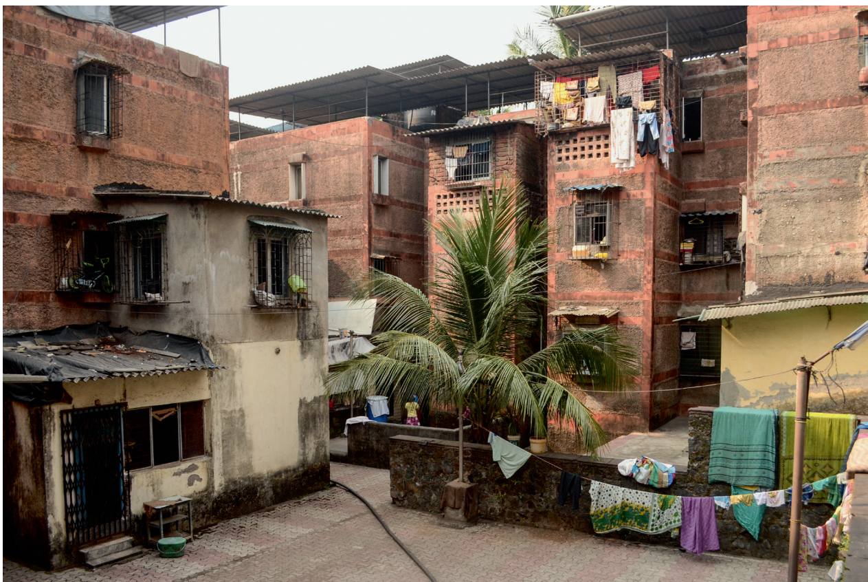
Woningen in cluster A1/B1/C1. Bewoners hebben hun leefruimte uitgebreid op daken en terrassen. Dwellings in cluster A1/B1/C1. The inhabitants have built extensions on the terraces and roofs.
