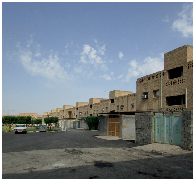
Gestapelde woningen (type 3) langs de openbare tuin Stacked dwellings (type 3) along the public garden
