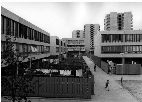
Laag- en hoogbouwblokken, Thamesmead, 1970 Low-rise and high-rise housing, Thamesmead, 1970
