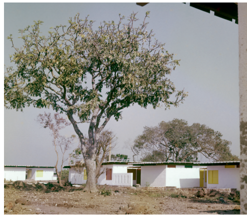
Type A woningen, Fria New Town, voorzijde Type A houses, Fria New Town, public side
