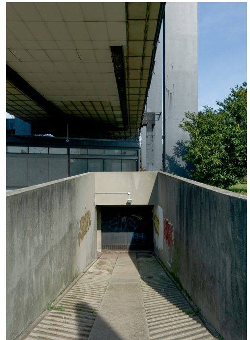
Entree kelderverdieping Entrance basement level
