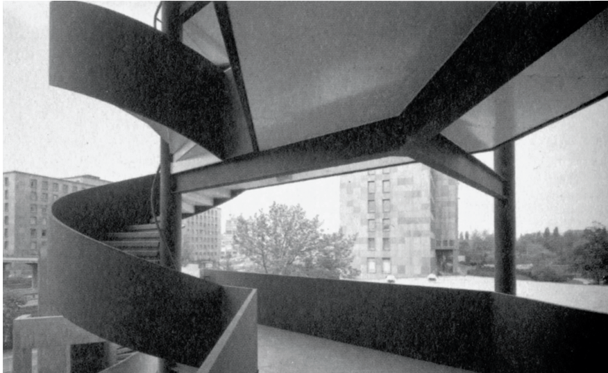
Bordes en trappenhuis Landing and staircase
