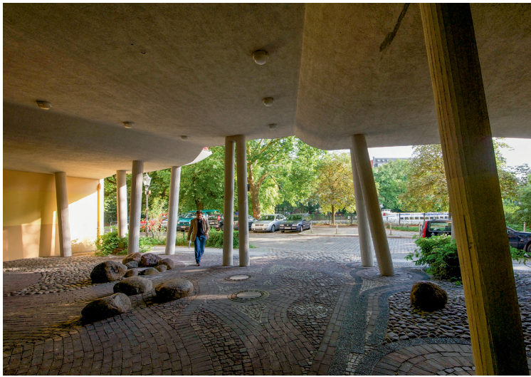
Onderdoorgang vanuit de binnentuin richting Fraenkelufer Underpass connecting the courtyard to Fraenkelufer
