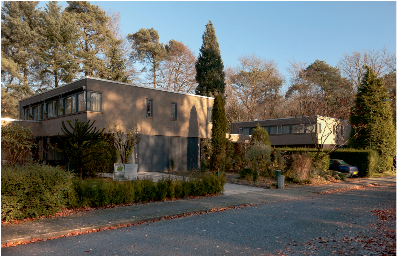
Zuidgevel prijsvraagwoning type Oost-West South façade of the 'Oost-West' design, from the competition
