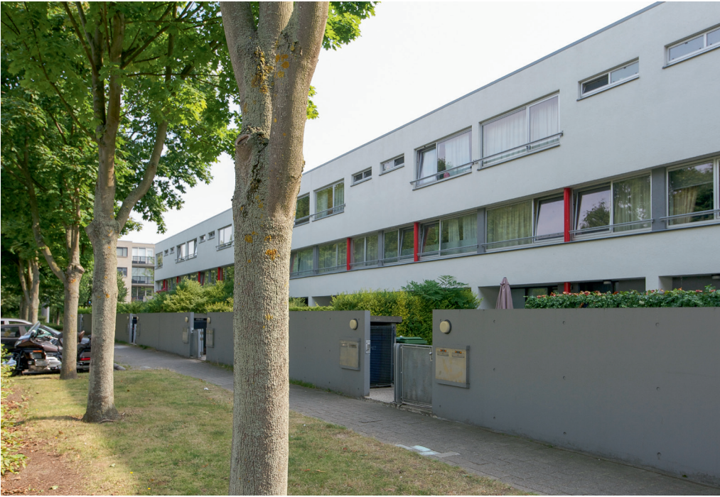
De woningen van Mecanoo Architecten, 2013 The dwellings by Mecanoo Architecten, 2013
