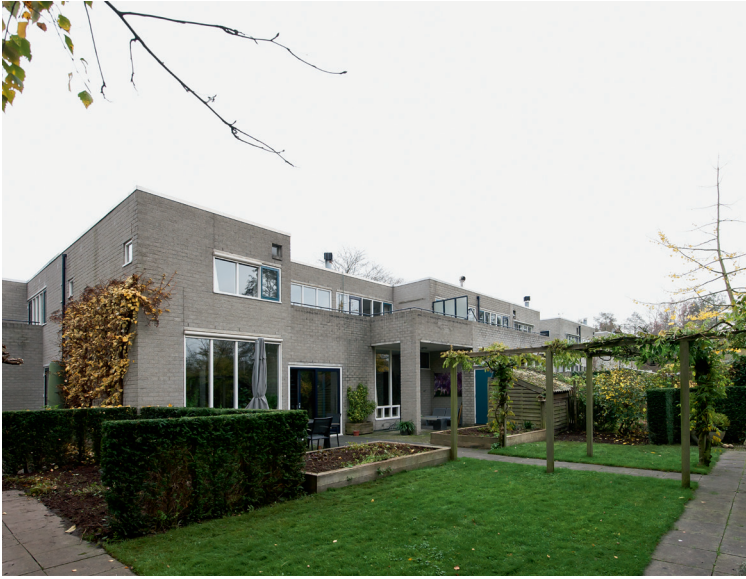
Achterzijde woningen Rear side of the houses
