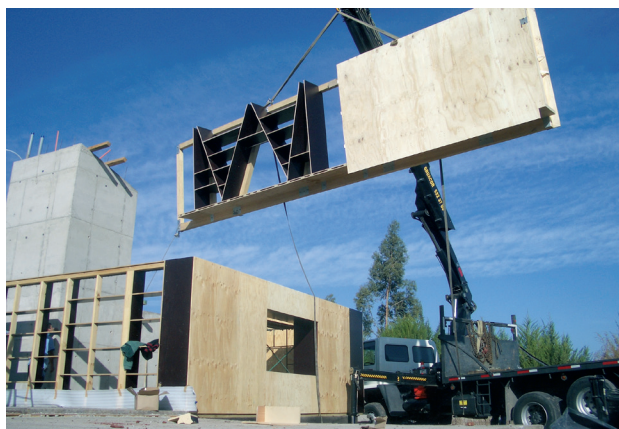
Inhijsen van de kastenwand Hoisting the wall unit into place
