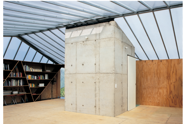
Betonnen kern met badkamer Concrete core with bathroom
