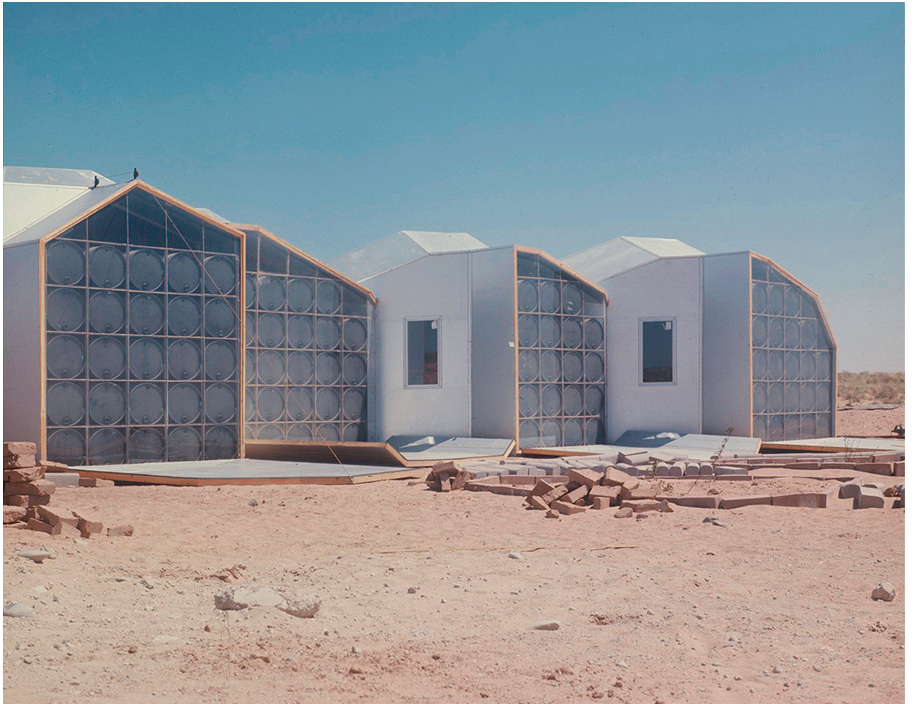
De drum walls (ca. 1972), met watergevulde olievaten The drum walls (circa 1972) of water-filled oil drums
