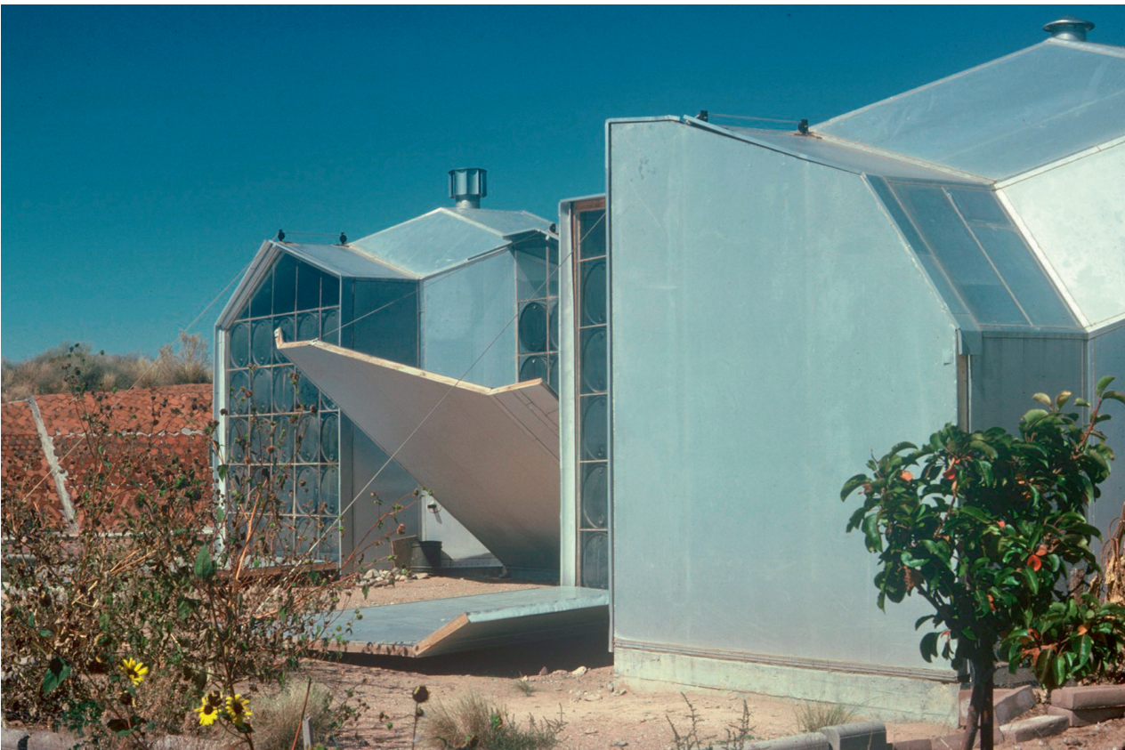
Drum wall met reflectiepanelen in open, halfopen en dichte toestand (ca. 1974) Drum wall with reflecting panels in open, half-open and closed position (ca. 1974)
