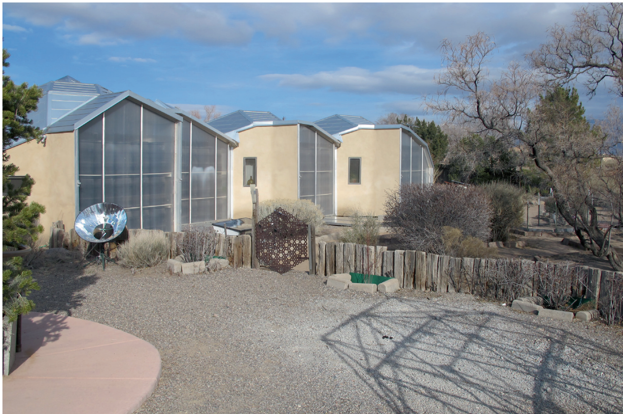
De huidige drum wall is beglaasd met Exolite acrylpanelen The current drum wall is glazed in Exolite acrylic panels
