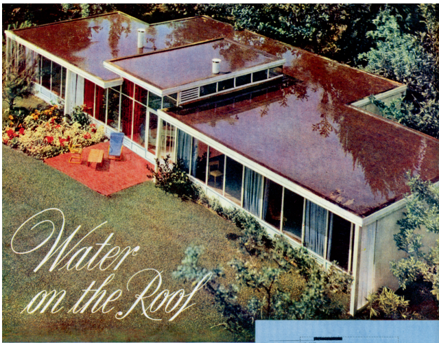
The water film helps to cool it in summer, the sun to warm it in winter.
