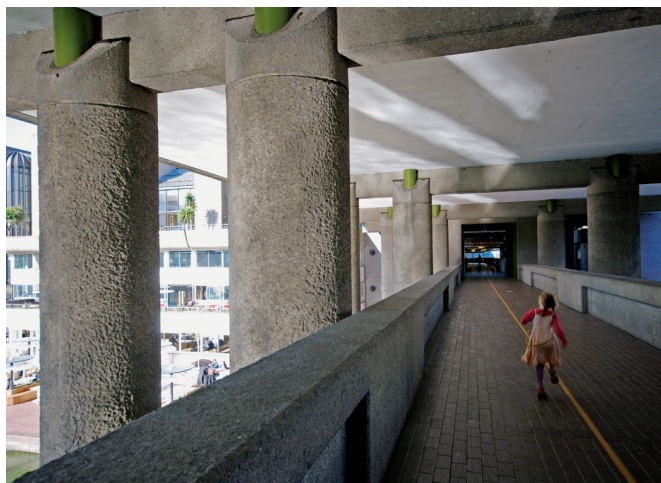
Passage op deckniveau over het water richting Arts Centre Passage at deck level over the water in the direction of the Arts Centre
