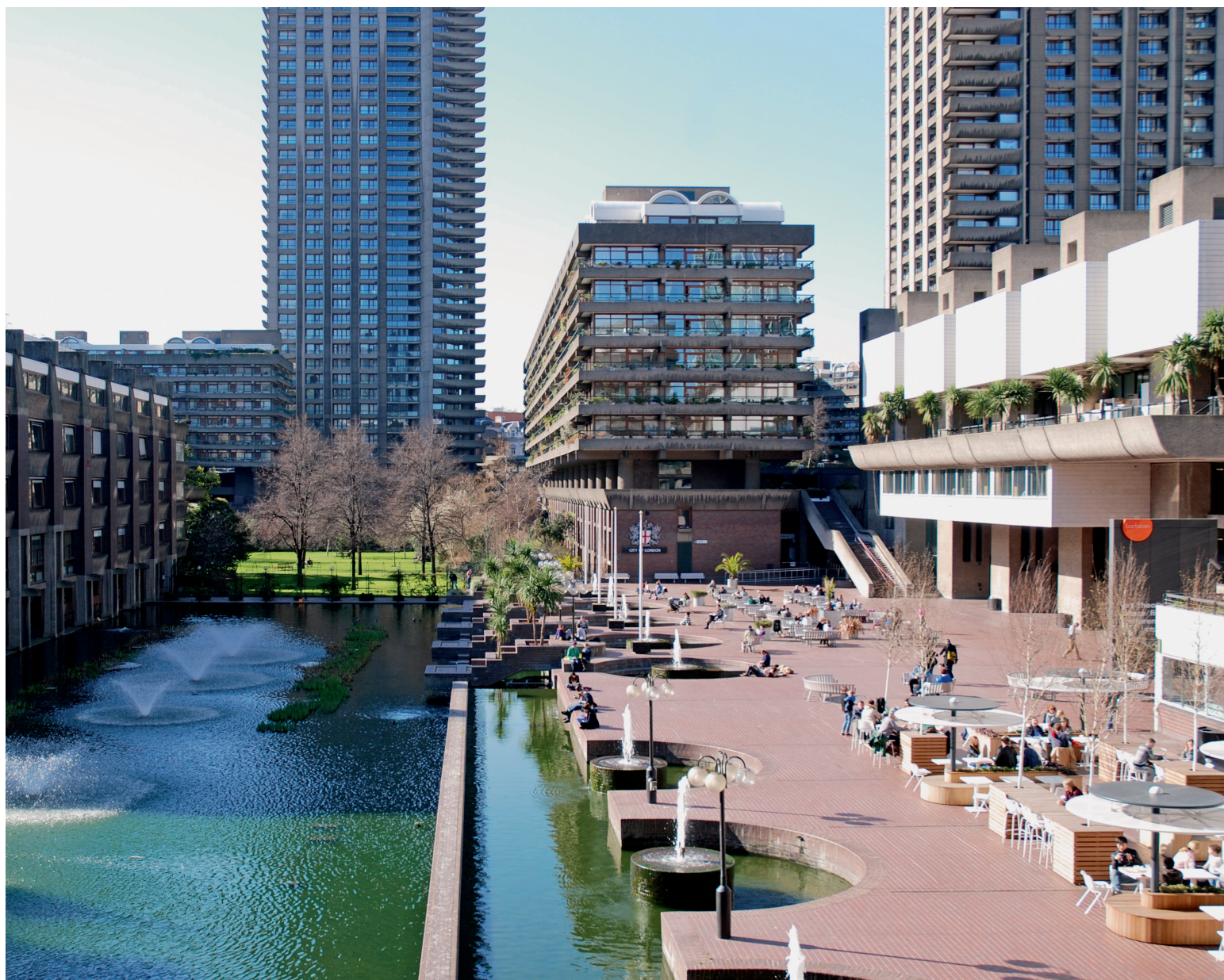
Centrale waterpartij met rechts het Barbican Arts Centre en links de City of London School for Girls Central water feature with, right, the Barbican Arts Centre and, left, the City of London School for Girls
