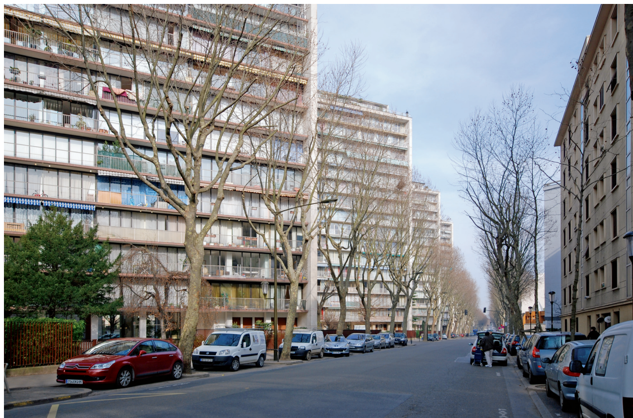
Woonstoren parallel aan de Seine, avenue Pierre-Grenier Residential towers parallel to the river Seine, avenue Pierre-Grenier
