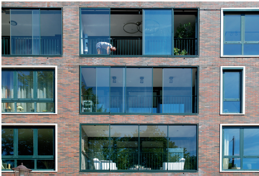
Gevelfragment Close-up of the façade
