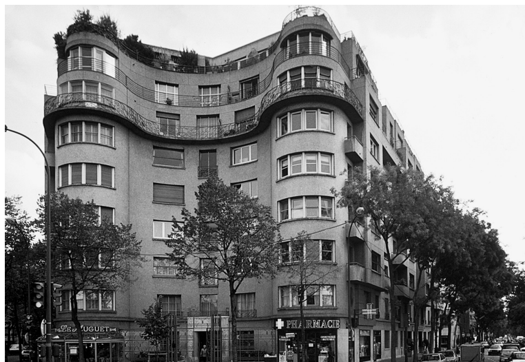
Gevel appartementengebouw Mirabeau-rotonde, Parijs; Bas-sompierre, De Rutté en Sirvin architectes, 1930-1933 Façade of apartment building on the Mirabeau roundabout, Bassompierre, by De Rutté and Servin Architects, 1930-1933
