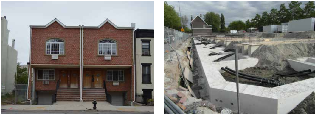
FIGURE 4.12 Left: wet-proofed two-family homes in Red Hook, New York City, US. Photo by author. Right: wet-proofed buildings at the Oranjeboomstraat, Feijenoord Rotterdam during construction. The hall is located at street level, while the ground floor is elevated above expected flood levels Photo by Eric Offereins on Skyscrapercity.com.
