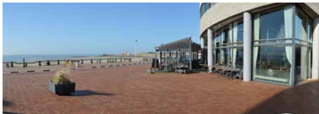
FIGURE 4.21 Convertibility. Providing high floor-to-ceiling height in the design of waterfront high-rise at the Vlissingen Boulevard (top picture) allows for a relative easy conversion of the first floor use in anticipation of an expected elevation of the boulevard in the future. Cross sections: Gemeente Vlissingen, 2012. Photo by author
