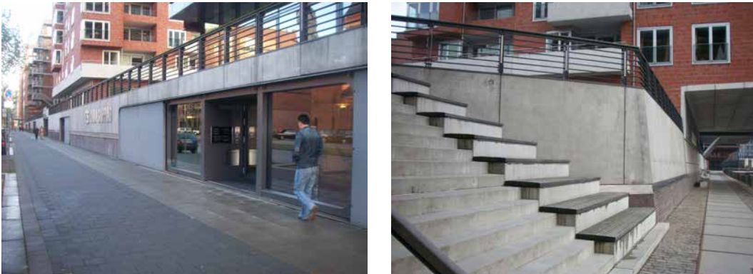
FIGURE 4.19 Hafencity in Hamburg (Germany) is an example of the robust design principle. In this new waterfront development flood protection is integrated into the architecture of buildings and urban design: all buildings are built on elevated flood proofed plinths that are used for parking and storage of 7.5 to 8.0 meter above mean sea level. This is 0.75 – 1.25 m above the highest storm surge ever recorded. Pictures by author.
