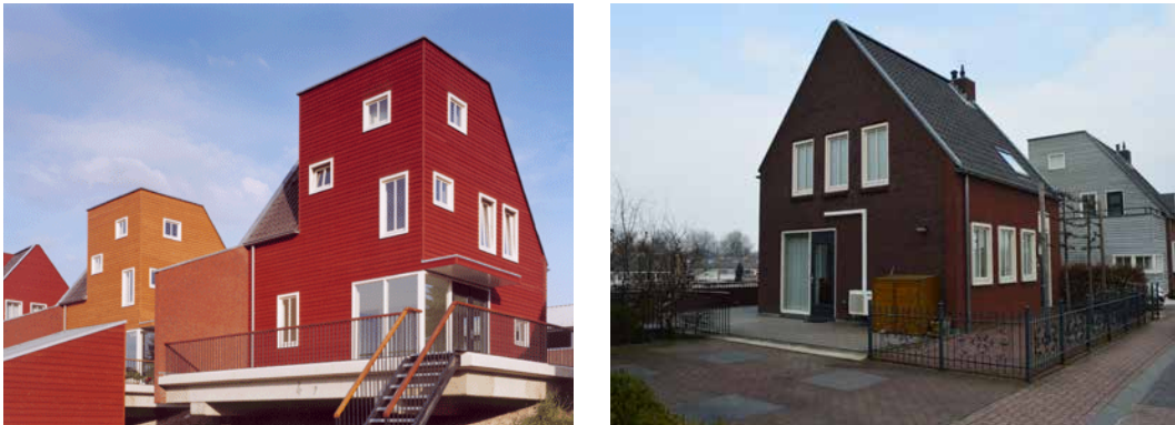
FIGURE 4.20 Adjustability. One-family homes at the Visschersbuurt at Papendrecht. The design of this row of buildings includes structural provisions to allow for a future elevation of the levee. The houses are constructed on a concrete floor slab resting on steel cylindrical pillars that can be raised to required elevation levels. Photo left courtesy of Kingma Roorda Architects, right photo by author.
