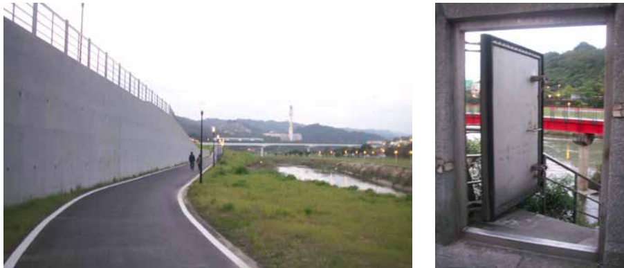
FIGURE 4.5 Floodwall along the Jingmei river in Taipei, Taiwan. Right picture: floodgate providing access to the waterfront park of one of Taipei’s urban rivers. Photos by author.
