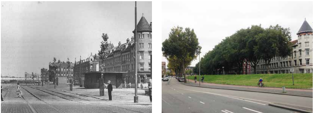
FIGURE 1.1 Reactive adaptation. Pictures show the Brede Hilledijk, Rotterdam in 1954 (left) and 2016 (right). In response to the 1953 flood a levee and floodwall was constructed that changed the form and function of the street and forms a major physical barrier between two neighbourhoods. Left picture RotterdamO10.nl. Right picture: by author.
