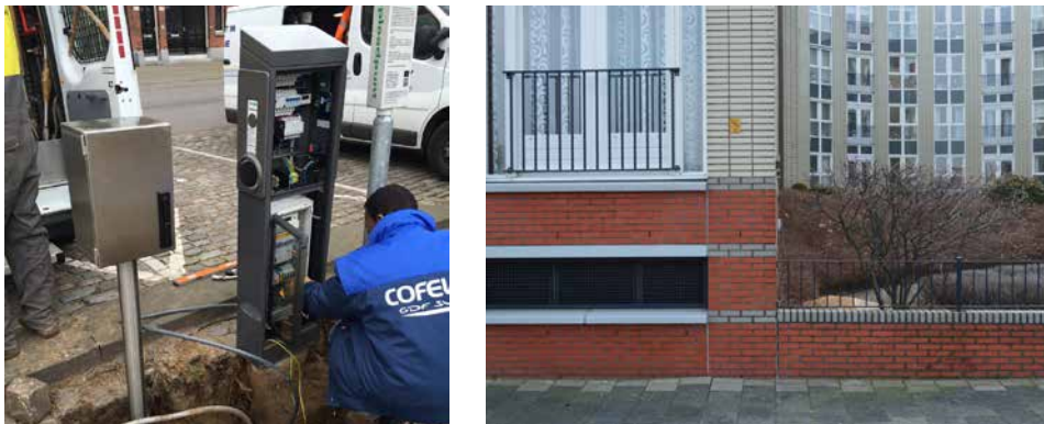
FIGURE 6.8 Left: retrofitting flood resilience to a charging post for electrical transport at the Noordereiland. Right: apartment building in Dordrecht built on a wet proofed semi below surface parking garage. Photo left: Gemeente Rotterdam, photo right by author.
