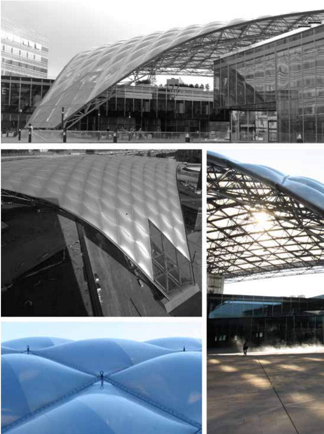
Figure 80 Images of the project. (Courtesy of Open Project Office and Ing. Giovanni Berti, copyright holders).
