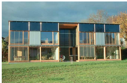
FIGURE 6.16 The sun-facing façade is almost completely transparent. Semi-detached passive houses in Bregenz, Austria by Walter Unterrainer. Reprinted from Walter Unterrainer Architektur Atelier website.
