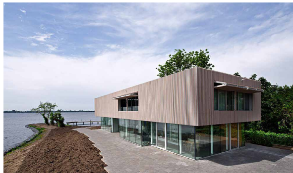
FIGURE 6.46 Folding shading device that forms an overhang; Villa Röhling, Kudelstaart, the Netherlands by Paul de Ruiter. Photo by Pieter Kers.
