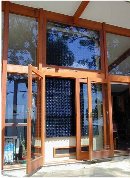
FIGURE 6.22 In a single-family house a Trombe wall is applied in lightweight structures and PCM modules are fixed to the back wall to add 'thermal mass'. The glass layer can be opened to flush the air cavity and prevent overheating in hot periods. Norton Summit 1, Adelaide, Australia by John Maitland. Reprinted from Energy Architecture website.
