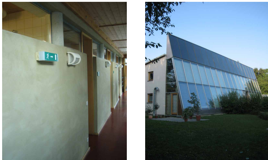
FIGURE 6.11 Thermal mass wall made of loam in AEE INTEC office building, Gleisdorf, Austria.
