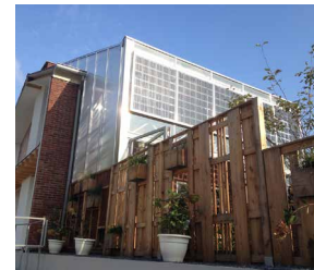
FIGURE 6.27 Sunspace in renovation, Prêt-à-loger house, entry of Delft University of Technology for the 2014 Solar Decathlon.
