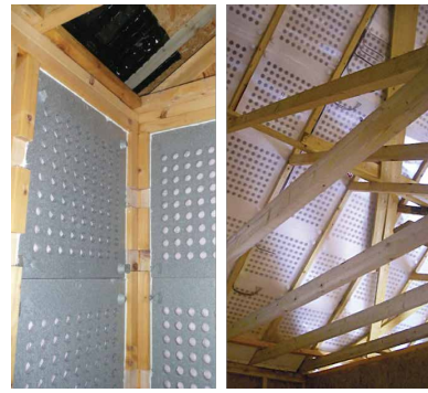
FIGURE 6.6 Modular dynamic insulation panels mounted in unfinished wall and roof structure. Reprinted from Energyflo Construction Technologies website.
