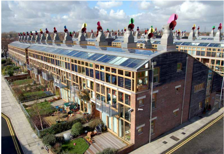
FIGURE 6.60 Rotating wind cowl that draws fresh air in and removes stale air at the same time. The system is equipped with a heat exchanger unit; BedZed, Hackbridge, London, United Kingdom by Bill Dunster. Photo by Tom Chance. Copyright: BioRegional.
