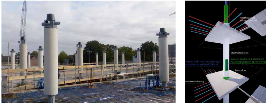
FIGURE 5.12 First application of energy columns in the new Stedelijk Gymnasium in Utrecht, the Netherlands by Thomas Rau. The energy column is developed in collaboration with JVZ and Grontmij. Reprinted from RAU (2009).
