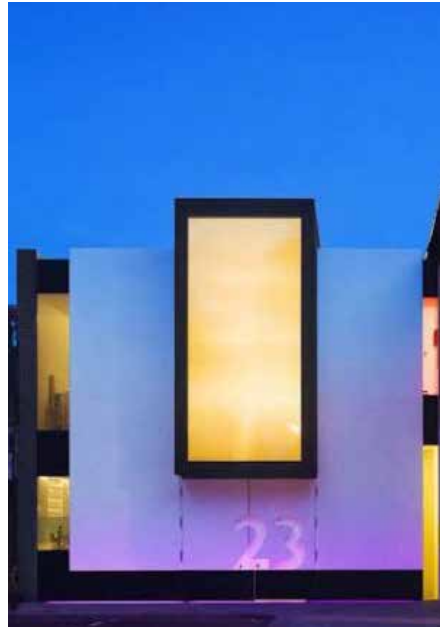
FIGURE 6.41 Double glazing unit with a Polymer dispersed liquid crystal (PDLC) layer that can be switched between a clear, transparent state and a frosted, opaque state. Reprinted from Intelligent Glass website.
