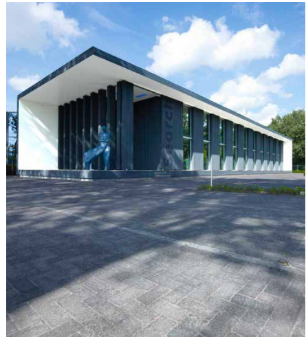
FIGURE 6.3 External folded thermal shutters. Search office building, Amsterdam, the Netherlands by Witteveen architects. Photo by Jeroen Musch.
