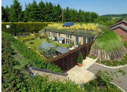
FIGURE 6.32 Honingham Social Housing, United Kingdom by SEArch architects is constructed at surface grade with a bank of earth bermed to its outer walls. Reprinted from SEArch architects website.
