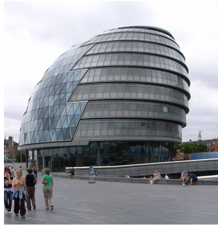
FIGURE 6.51 Each cantilevered storey acts as an overhang for the windows of the storey below; London Town Hall, London, United Kingdom by Norman Foster. Photo by Steve Cadman.
