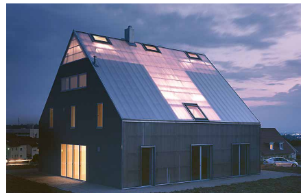
FIGURE 6.17 Transparent roof elements see supply direct solar gains in the common transfer space between the two dwellings. Patchwork-House in Müllheim, Germany by Pfeifer Roser Kuhn Architekten. Photo by Ruedi Walti.
