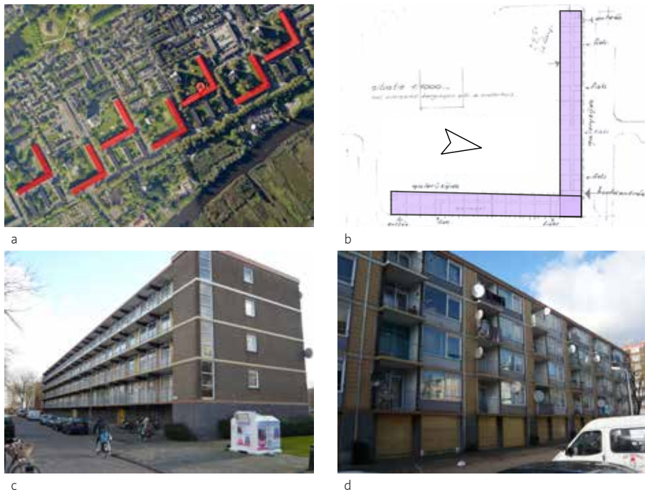
Figure 6.5 (a) Aerial view of Poelenburg district and (b) the L-shaped buildings (c) Gallery and (d) back façade. Image courtesy Edwin Tensen
