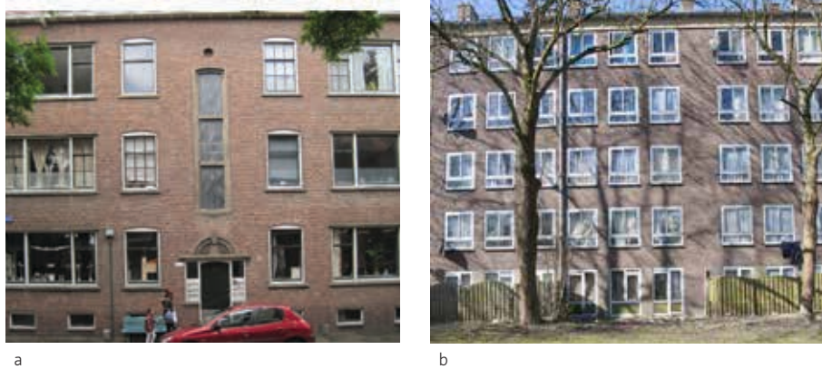
Figure 8.3 The apartment building with the masonry wall and single window (a) and cavity wall and double window
