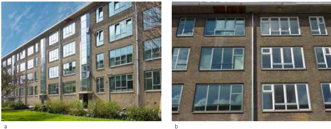
Figure 4.4 Renovation of Koningenvrouwen van Landlust in Amsterdam – Eigen Haard (Image source: courtesy of DeGroot en Visser, façade construction). The building was built in the 1930's and it is currently listed as a monument. The original steel framed windows had already been replaced with double-glazed windows in the 80's. However their performance was not sufficient, nor was the architectural quality, which was far from the original slim, steel profiles. For this reason a new system with a sightline of only 5 cm was developed to replace the windows. The system is highly insulated with an U_f=1.93 \text{ W/m}^2\text{K} . The windows are structural glazed to be able to use a single sightline. There was a special coating applied with a steel look and twinkle. The window replacement was coupled with the application of internal insulation.
