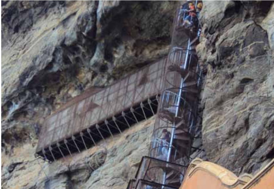
Figure 3.13 Spiral staircases installed to view the surviving paintings
