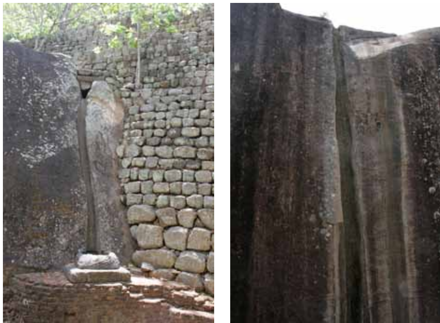
Figure 5.73 Rock-cut vertical drains on the rock boulders of the hilly terrain
