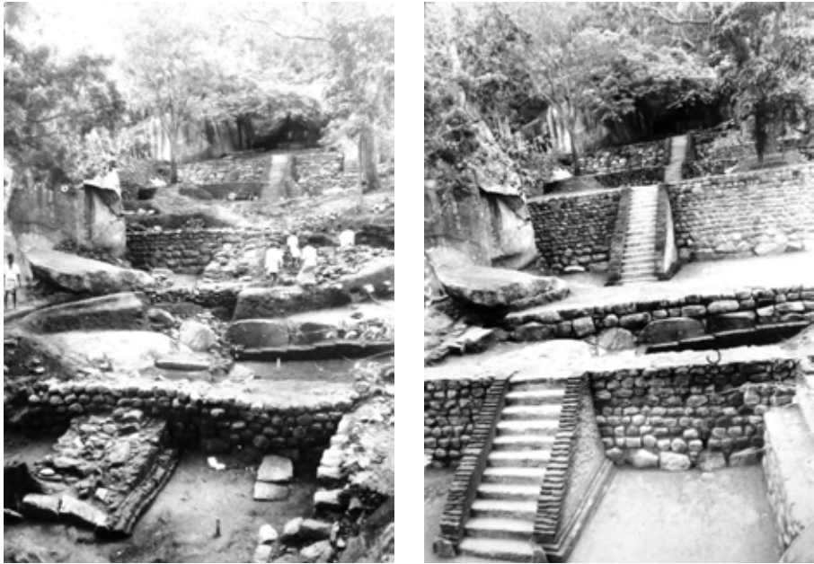
Figure 3.12 Western route through the hilly terrain leading up to the Boulder Arch No. 1, after excavations and after conservation (courtesy: Central Cultural Fund)
