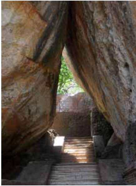
Figure 2.23 Boulder arch No. 01
