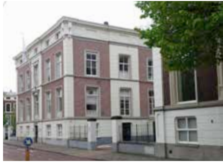
1 Alexanderstraat, architect Delia
