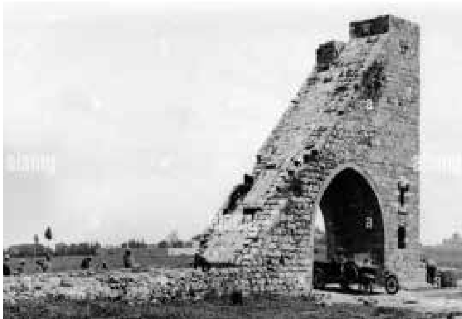
FIG. 5.6 A view of the Syphon Aqueduct over the Acre Sidon Road. B01306_Alamy
