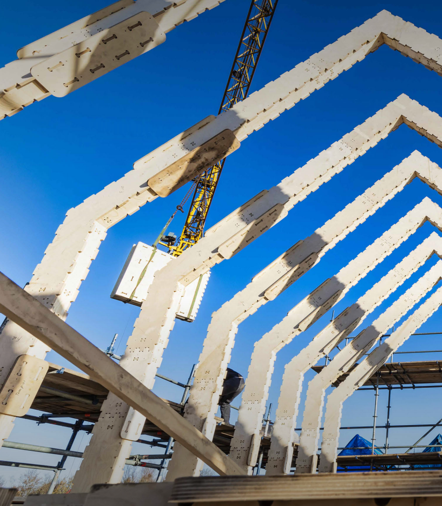
The construction of a Wikihouse in Almere in the Netherlands as part of the Housing 4.0 Energy (H4.0E) project funded by Interreg North-West Europe. Copyright: Wikihouse.
