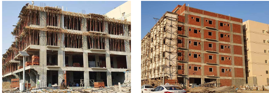
FIG. 3.10 20 centimetres blocks for wall-filling within the skeleton structure.
