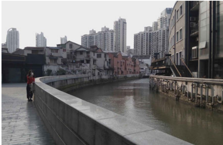
FIG. 3.5 Most creeks disappeared and the few remaining ones, such as Hongkou Creek, are often disconnected from urban life by floodwalls (photo by author, 2018).
