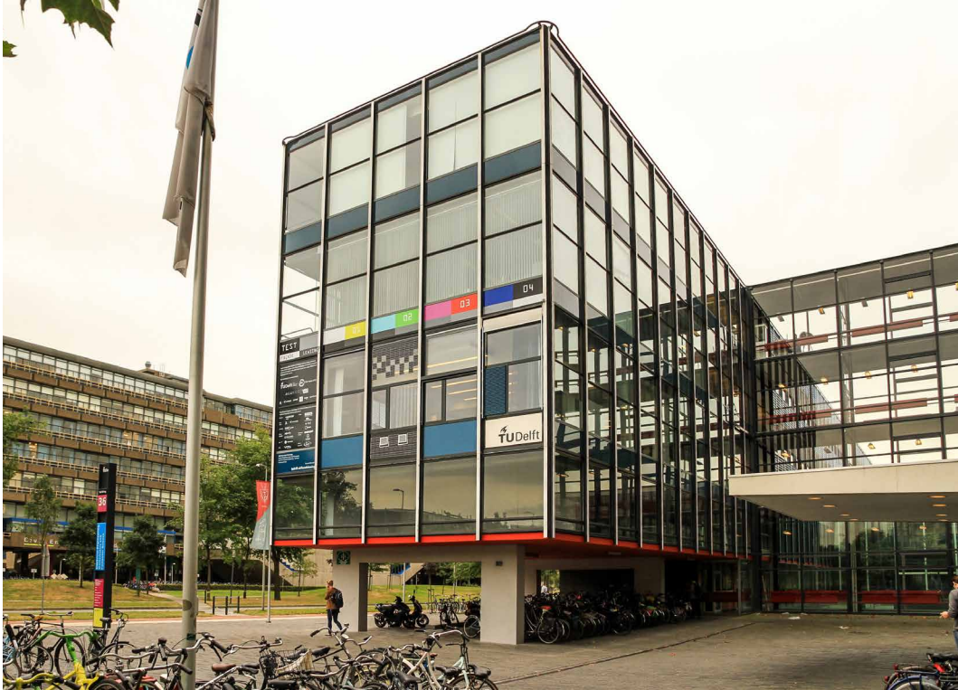
FIG. 4.1 Photograph of the completed “Façade Leasing Pilot Project” at TU Delft’s EWI faculty building (Photo: Marcel Bilow, 2016)
