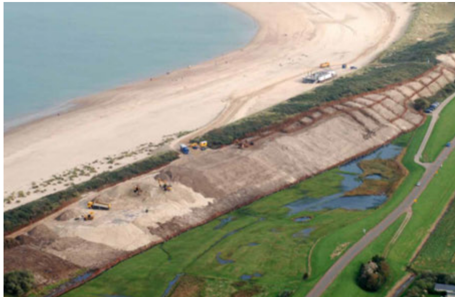
FIG. 3.10 Dune reinforcement at Renesse, Netherlands (2014). Source: Sinke Group.
