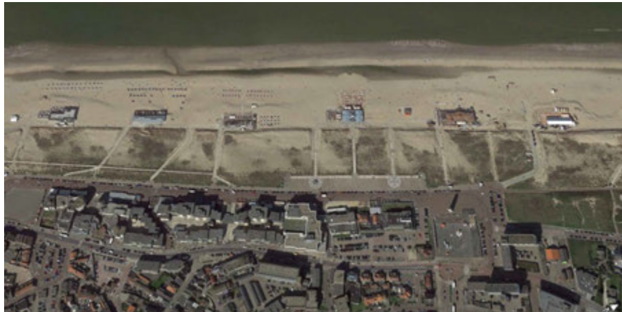
FIG. APP.A.15 Aerial photograph of the Noordwijk beachfront with sand deposition in the dunes, caused by beach buildings and accesses, April 2018. Source: Google Earth.
