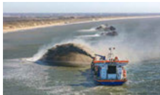
FIG. 2.7 Shoreface nourishment in North Holland, NL 2020 (middle). Source: Rijkswaterstaat.
