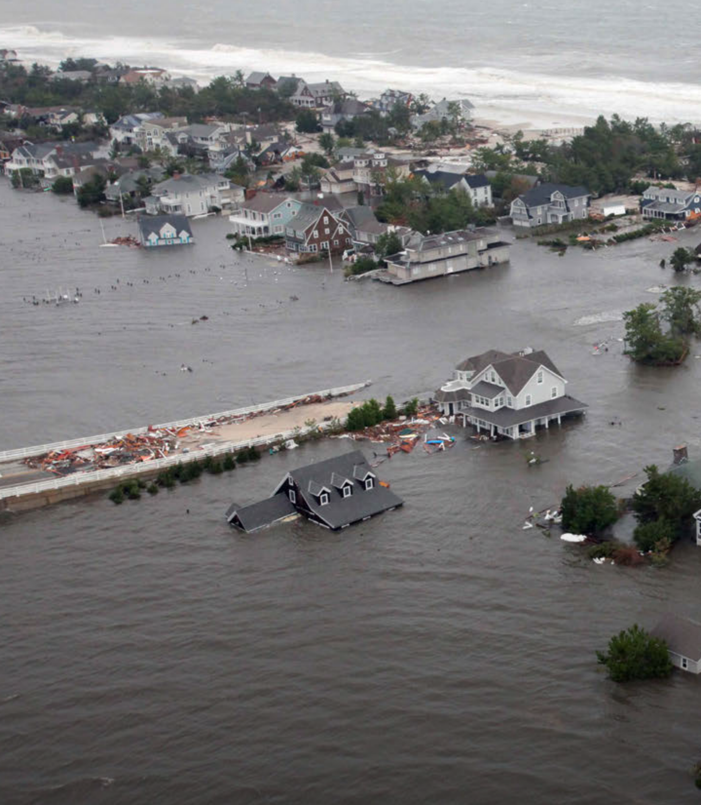
Aerial view of the damage caused by Hurricane Sandy to the sandy urbanized New Jersey coast (October 2012). Source: National Guard of the United States.
