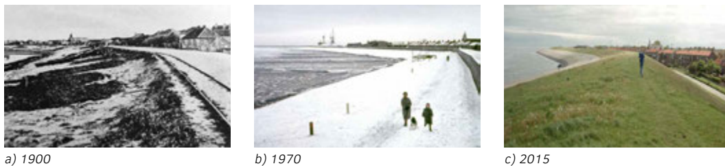
FIG. 1.3 The seawall at Den Helder in 1900 (left), 1970 (middle) and 2015 (right). Due to coastal reinforcement, the seaside setting of the fishing village was disrupted over time, cutting the town off from the sea with a 12m-high sea wall. Sources: E. de Jong (middle) and Rijkswaterstaat / Simon Warner (right).
