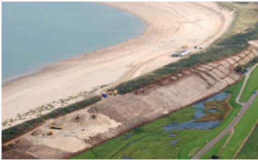
FIG. 2.9 Dune reinforcement in Renesse, NL 2014 (left). Image by the Sinke group.
