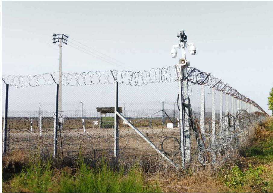
FIG. 4.2 The Hungarian border fence in the proximity of Rabe village (Serbia), September 2020. Source: photo by author.
