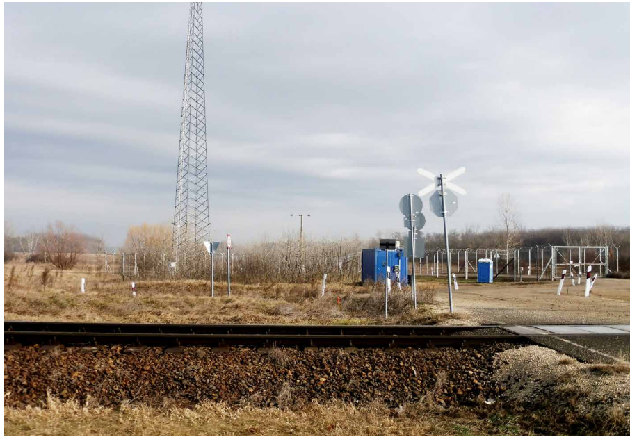
FIG. 4.18 The double line of fencing is interrupted to allow the passage of the railway in the proximity of Kelebia (Hungary), January 2022. Source: photo by author.
