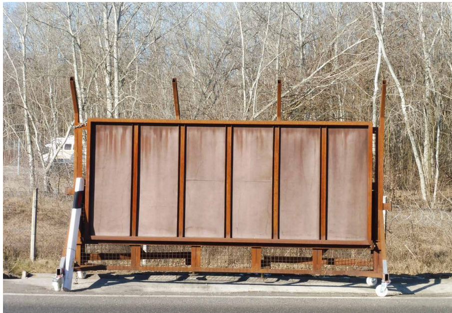
FIG. 4.5 Mobile metal border closures that were temporarily used to stop the arrival of migrants in 2015, Röszke (Hungary), January 2022. Source: photo by author.
