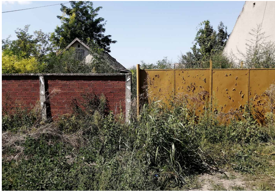
FIG. 5.16 View of the village houses from the main road. Majdan (Serbia), September 2020. Source: photo by author.
