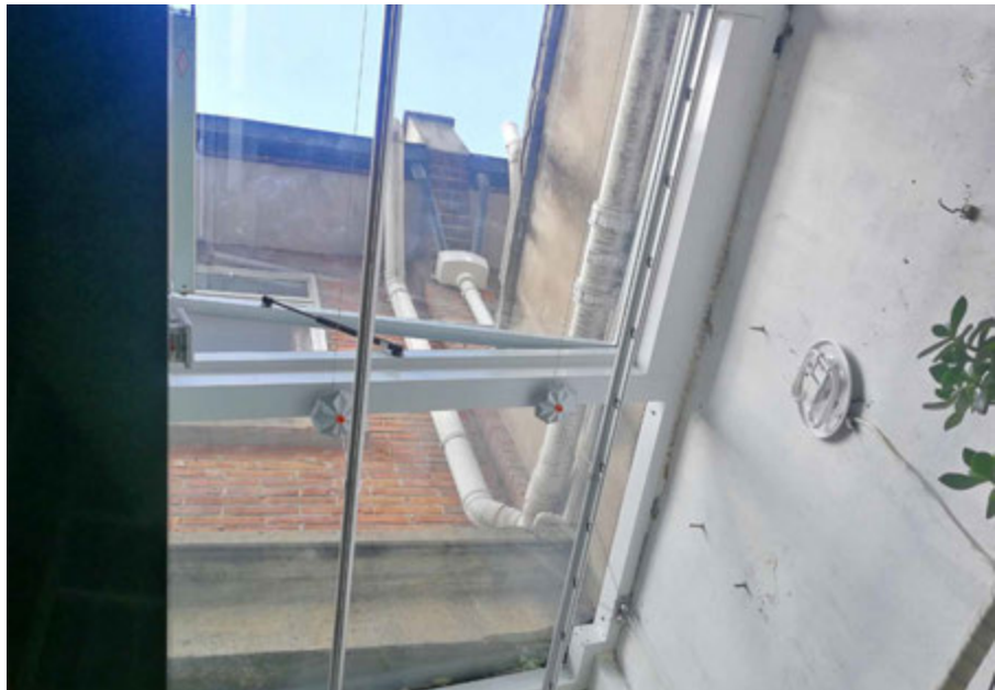
FIG. 8.25 The added transparent roof in the original courtyard place of Bugaoli No. 59, for cloth washing and cooking. Source: author, 2018.
