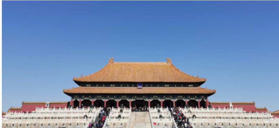
FIG. 3.5 The hip roof with double eaves is the highest form of roofing style in China's ancient architecture. This roof style is applied to Hall of Supreme Harmony (Taihe Dian, 太和殿), the largest hall in the Forbidden City, to reflect imperial power. Source: author, 2019.
