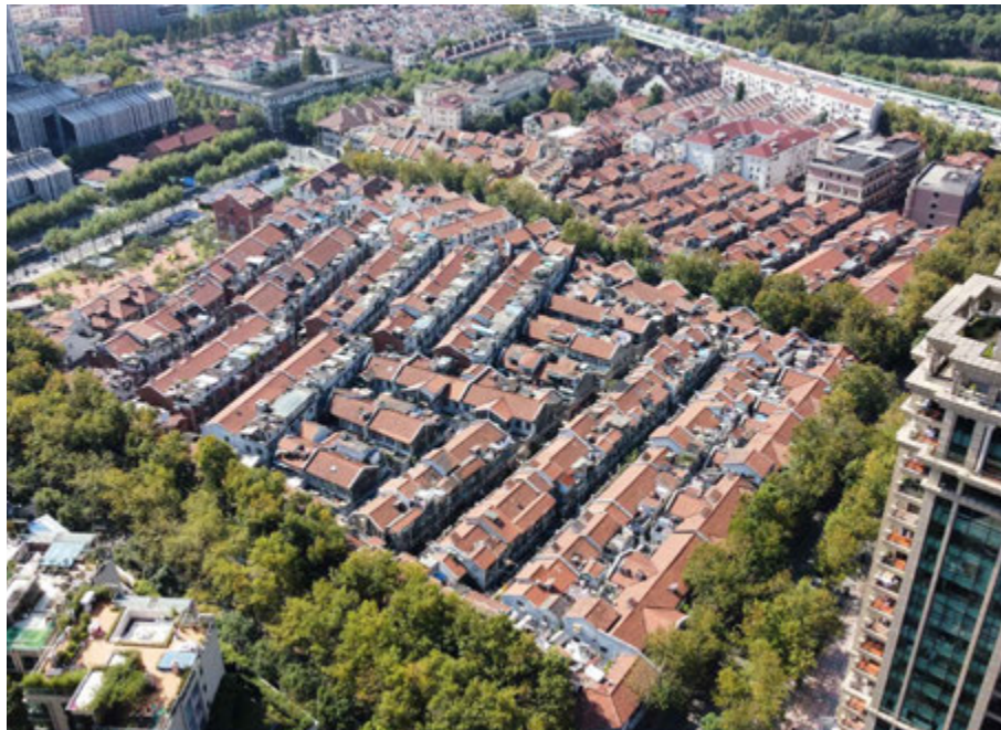
FIG. 6.27 The historic lilong neighbourhoods Xichengli (西成里), South Puqingli (普庆里) and more to the southwest side of Xintiandi, across Madang Road and, surrounded by high-rises and other contemporary architecture for commercial interests. Source: author 2021.
