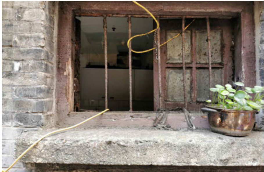
FIG. 7.24 A decaying timber window frame and stained and rusted window grilles on the façade of a lilong residence. Source: author, 2021.
