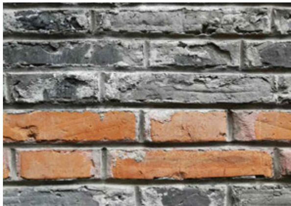
FIG. 6.16 Conserved external brick walls with original architectural materials. Source: author, 2021.
