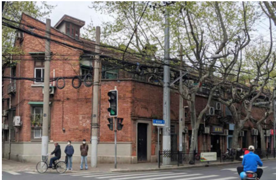
FIG. 8.7 The corner of Bugaoli at the crossroad of the South Shaanxi Road and the West Jianguo Road is built with cement-encrusted two-slope gable walls today, the stepped gables (matouqiang) are nowhere in sight today. Source: author, 2018.
