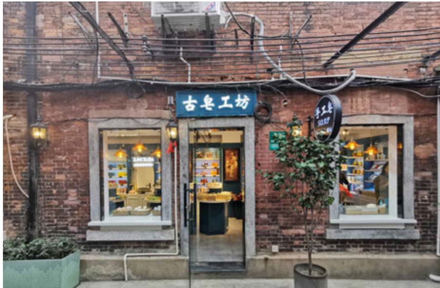
FIG. 7.21 Because of the demand for openness to the public, this handmade soap store opened one extra opening front door in the brick wall and consequently panned the original left window of the ground floor. Source: author, 2021.
