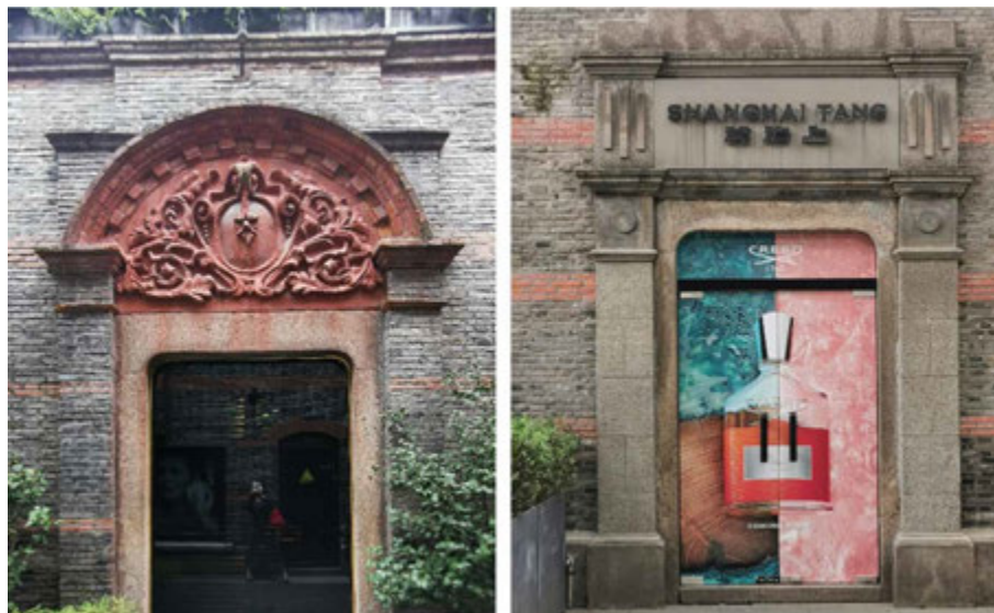
FIG. 6.9 Different curved stone or cement plastering pediments on architectural facades of buildings in Xintiandi after transformation. Source: author, 2021.
