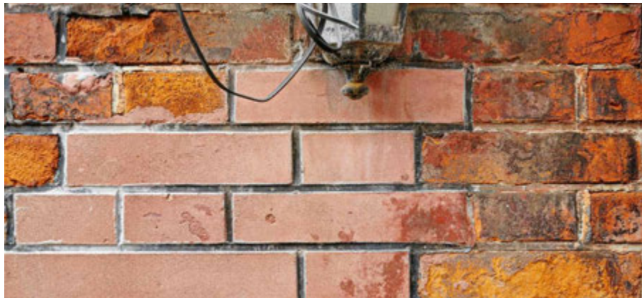
FIG. 7.22 The faked red brick wall with an additional layering of new tiles. Source: author, 2021.
