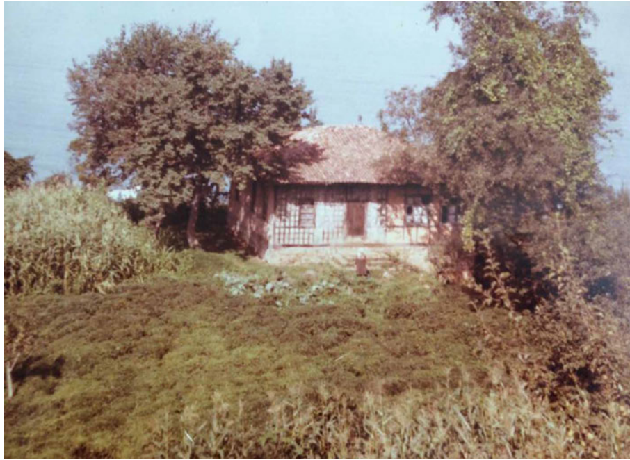
FIG. 2.4 A typical Lazuri house with its regular and modular form of façade which consists of small and rectangular frames filled with stones inside. Source: Laz, CC BY-SA 4.0 < https://creativecommons.org/licenses/by-sa/4.0/ >, via Wikimedia Commons
