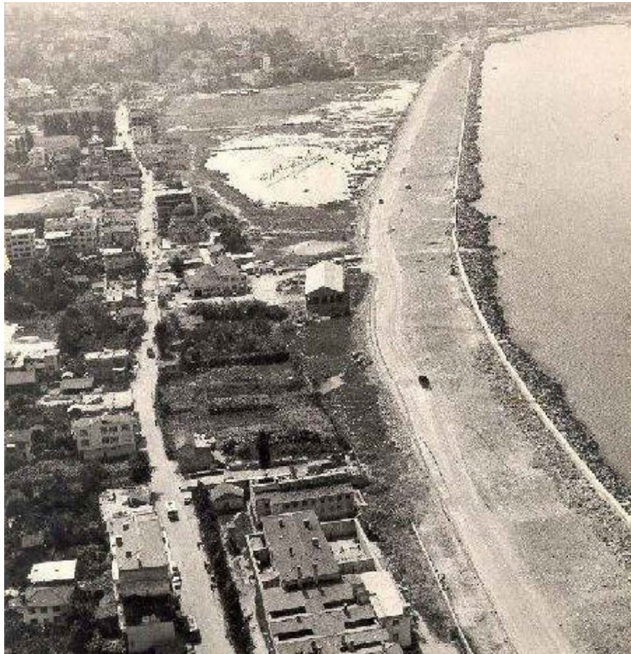
FIG. 5.2 The construction of the Black Sea coastal road 1960s in the city of Rize caused the irreversible destruction of seafront mansions. Source: https://www.tarihtarih.com/
