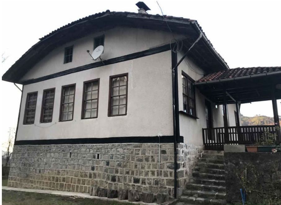
FIG. 6.18 Sevketybeyoglu building is majorly transformed with the opening of a terrace in the entrance and the plastering of the façade. Source: author.
