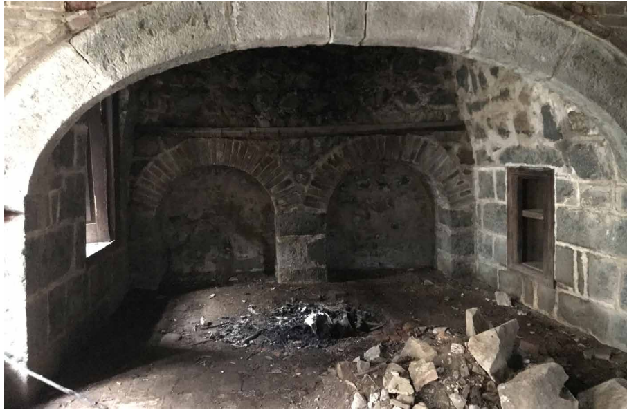
FIG. 3.19 There is a large bakery oven in the kitchen that connects to the brick chimney. Source: author.
