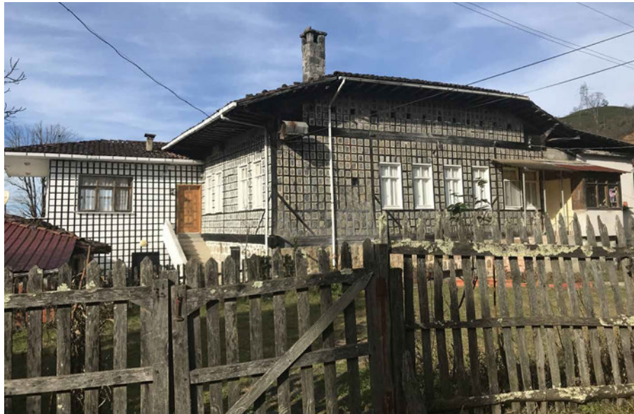
FIG. 6.16 One of the houses of 5 evler is renovated including the stairs, toilet, and an additional unit. Fındıklı Çağlayan Village 5 evler Parcel no 110 and 111. Source: author.
