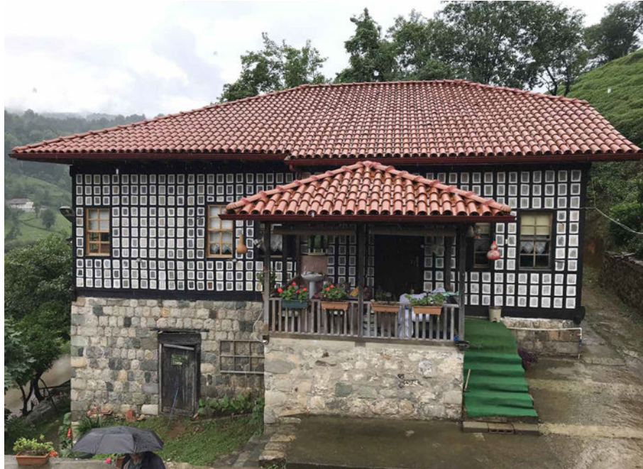
FIG. 6.10 The standalone window on the corner of the façade of the ground floor was accepted as original by the conservation architect. Source: author.
