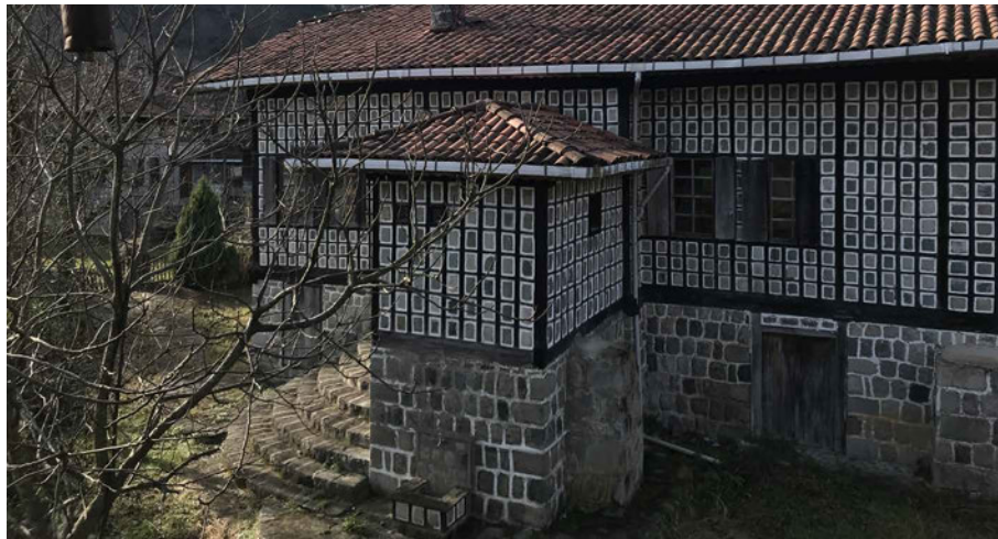
FIG. 4.7 The quarter-circle-shaped stairs reach the main entrance. There are irregularly placed windows in each timber frame. Source: author.
