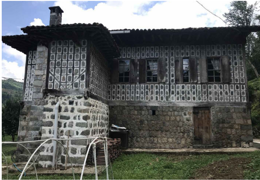
FIG. 3.25 Typical vernacular heritage in the region with a stone-infilled timber mansion. Source: author.
