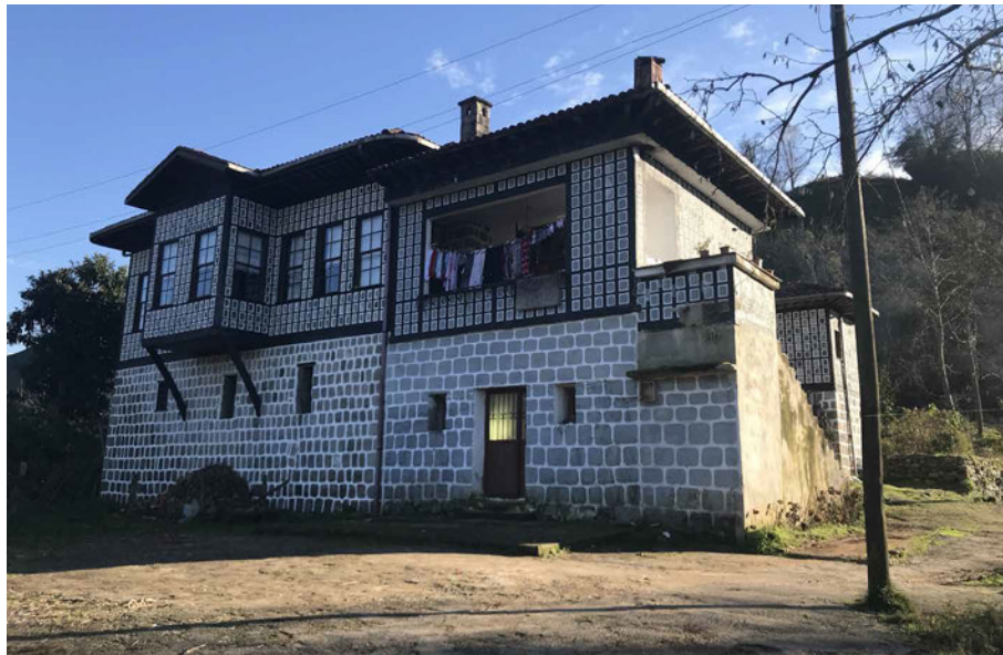
FIG. 6.5 The building, owned by the Okman household, was not only extended but also had improper units. A closed balcony with a wide opening is added in contrast to the bay window, which was constructed in line with the local climate in Çağlayan village. Source: author.
