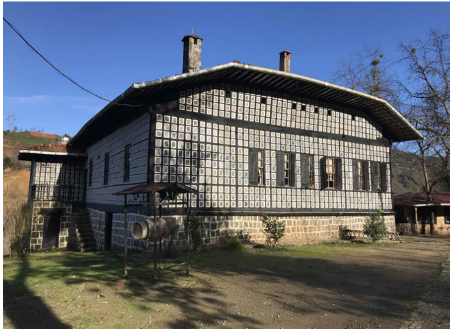
FIG. 4.14 The wooden shutters are not only placed on one façade. The façade on the opposite entrance to the main entrance has no wooden shutters as it does not receive enough sunlight. The arced shape roof though renovated extends widely. Unlike others, the building is located in a lowland. Source: author.
