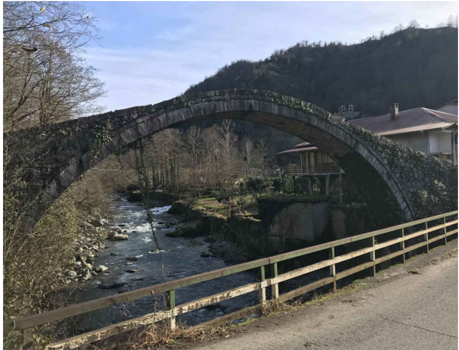
FIG. 3.28 Stone bridge in Çağlayan village. Source: author.
