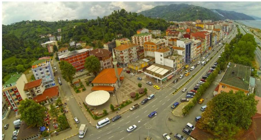
FIG. 3.12 The narrow strip of coastline, also known as the centre of the Fındıklı district is dense with rapid urbanization. The majority of public places such as mosques, public administration, education centre, library are located in this area. Source: Erkan Aksu Photography Archives.
