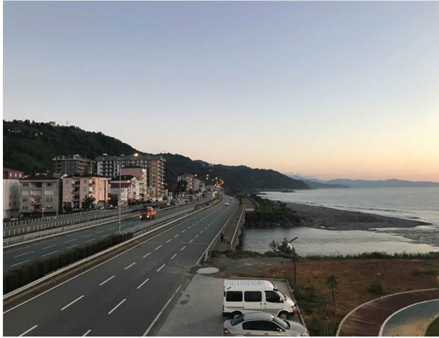
FIG. 5.11 The Karadeniz Sahil Yolu (Black Sea Seaside Highway) today with its two-way road cuts the coast as the district centre and the sea. Although now there is a public park for recreational purposes, the infrastructure is often flooded. Source: author.
