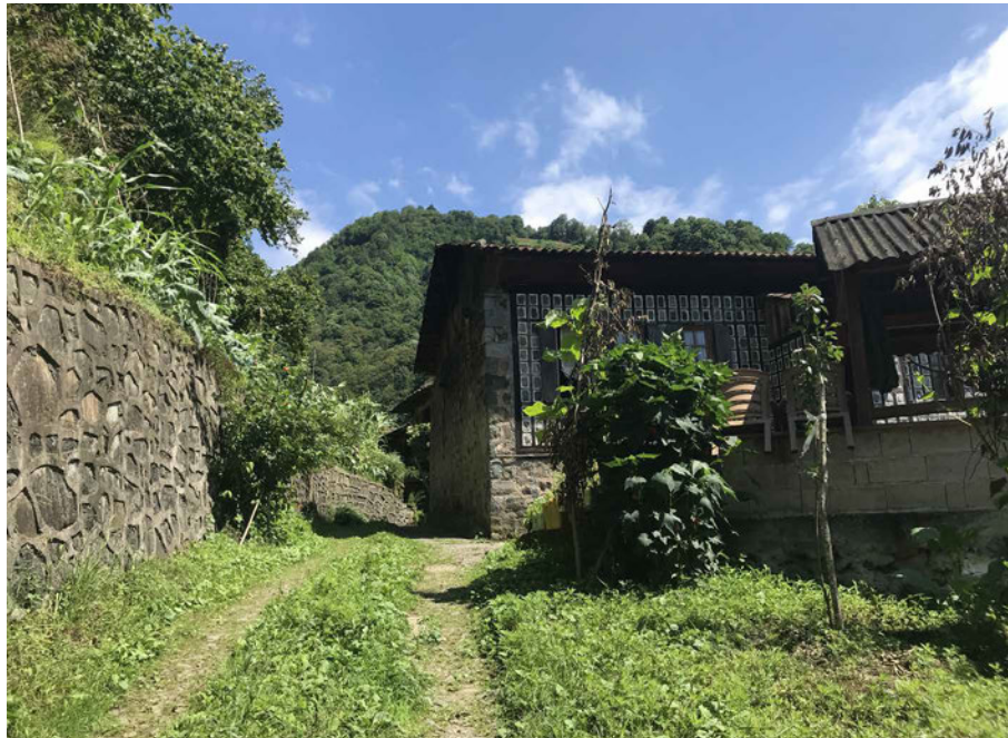
FIG. 7.8 T.H. house is vulnerable to rock falls, which is why the rear façade was built with stone with no openings. Source: author.
