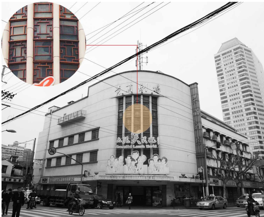
FIG. 8.4 Window Patterns of the Street Façade of the Huangpu Theatre. Source: Edited by Lu Li based on image obtained via Wiki Commons. 433
