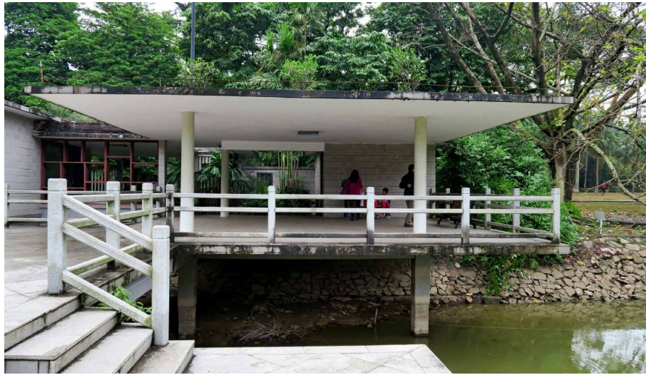
FIG. 8.6 The Water Pavilion in the South China Botanical Garden, Guangzhou. Source: im拓海. 439
