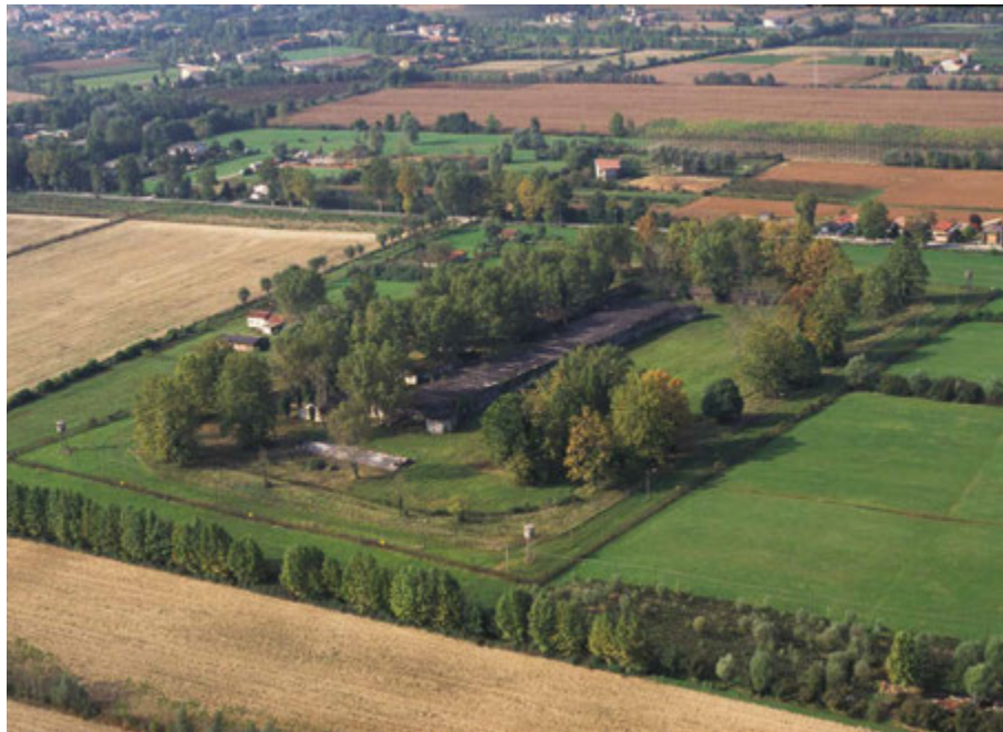
FIG. 5.81 Venice (IT), Forte Mezzacapo: aerial picture where the trace of the former moat surrounding the fort, now buried, is recognizable (Archive Associazione dalla Guerra alla Pace)
