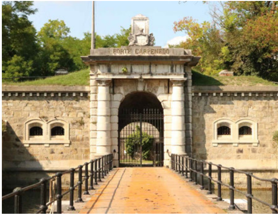
FIG. 5.69 Venice (IT), Forte Carpenedo: the main portal and the access bridge (F. Marulo 2020)
