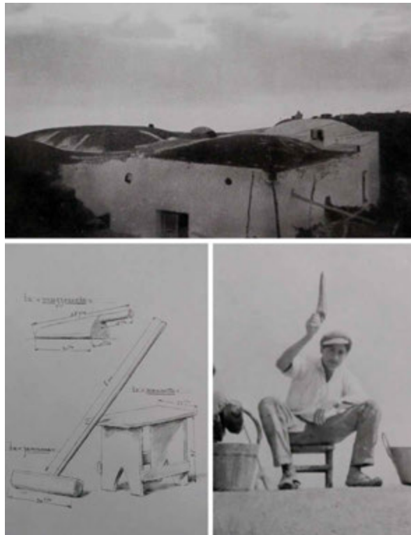
FIG. 3.10 Some of the images associated to E. Cerio's description of the landscape of Capri: the roofs of Anacapri (top); tools for 'beating' the roofs (below, left); worker handling the mazzoccola (mallet) (below, right) (Cerio 1923)
