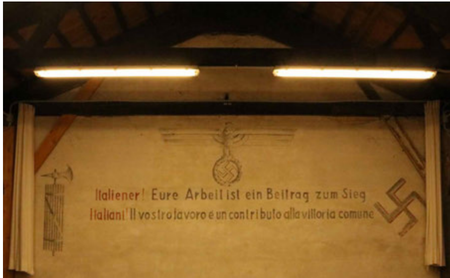
FIG. 5.76 Venice (IT), Forte Mezzacapo, shed 2 (former projectile workshop): nazi-fascist inscription after restoration (2011). Since the building is used for theatre performances, curtains are occasionally used to hide this difficult memory (F. Marulo 2020)
