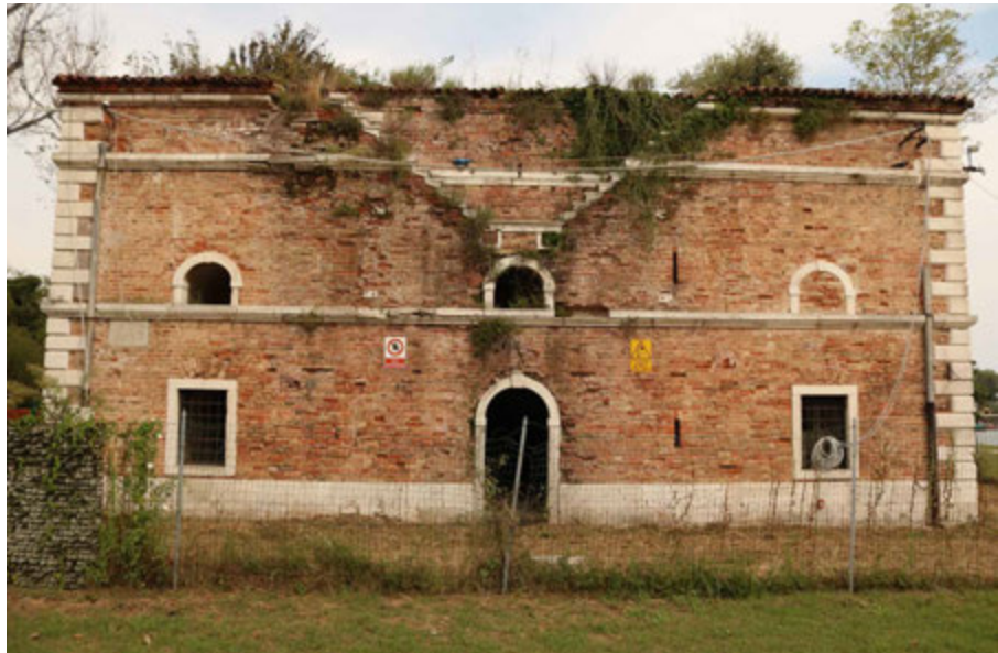
FIG. 5.52 Venice (IT), Forte Marghera: French barracks (8), western façade (F. Marulo, 2020)
