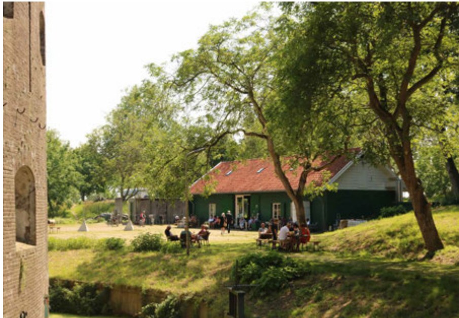
FIG. 4.97 Vijfheerenlanden (NL), Fort Everdingen: the wooden warehouse reused as a testing room for the brewery (F. Marulo 2019)
