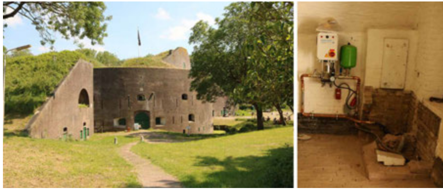
FIG. 4.98 Vijfheerenlanden (NL), Fort Everdingen: the water collection system of the tower building is reused in the brewing process (F. Marulo 2019)
