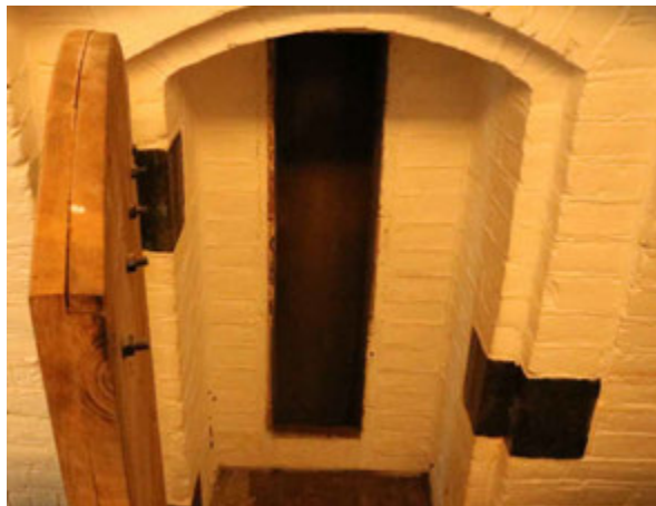
FIG. 4.74 Houten (NL), Lunet aan de Snel, bombproof barracks: the reuse of the water collection system (F. Marulo 2019)
