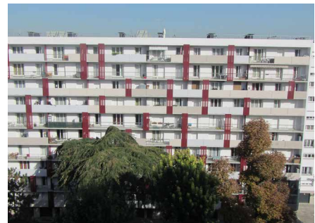
Vitry-sur-Seine project after renovation
