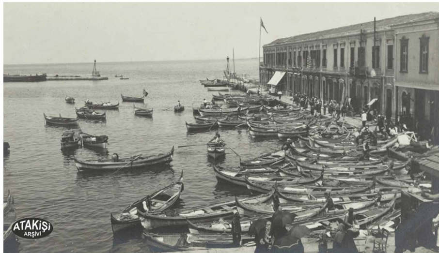
FIG. 6.2 Kayiks and Pasaport Building (courtesy of Tufan Atakışi).
