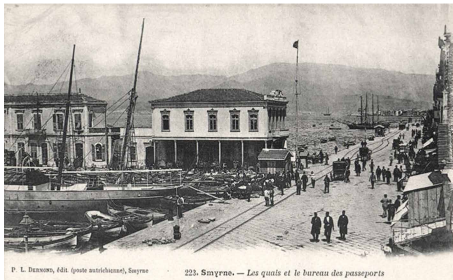
FIG. 5.1 Pasaport building and the quay (courtesy of Levantine Heritage Foundation).
