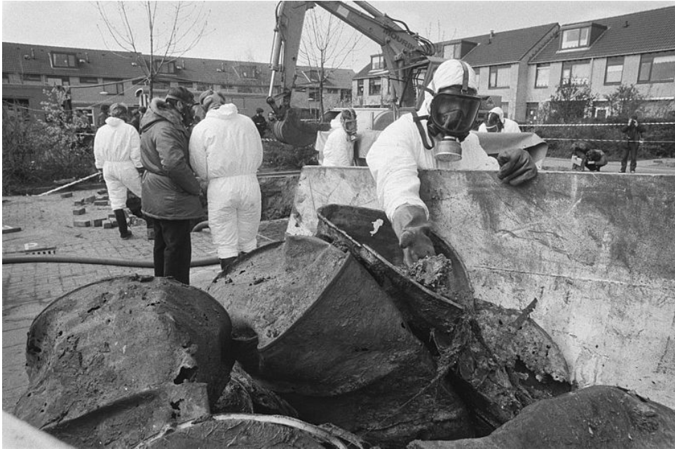
Figure 4.7: Barrels of chemical wastes are dug up in Lekkerkerk in 1980. Picture by Dijk, Hans van / Anefo. Source: Nationaal Archief, Den Haag, nummertoeegang 2.24.01.05, bestanddeelnummer 930-7893. Found on Wikimedia.
