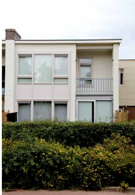
FIG. 7.34 A renovated north-east facing façade of an un-duplexed unit: the 'temporary' aluminium enclosing of the veranda is visible in the bottom right (2018).
