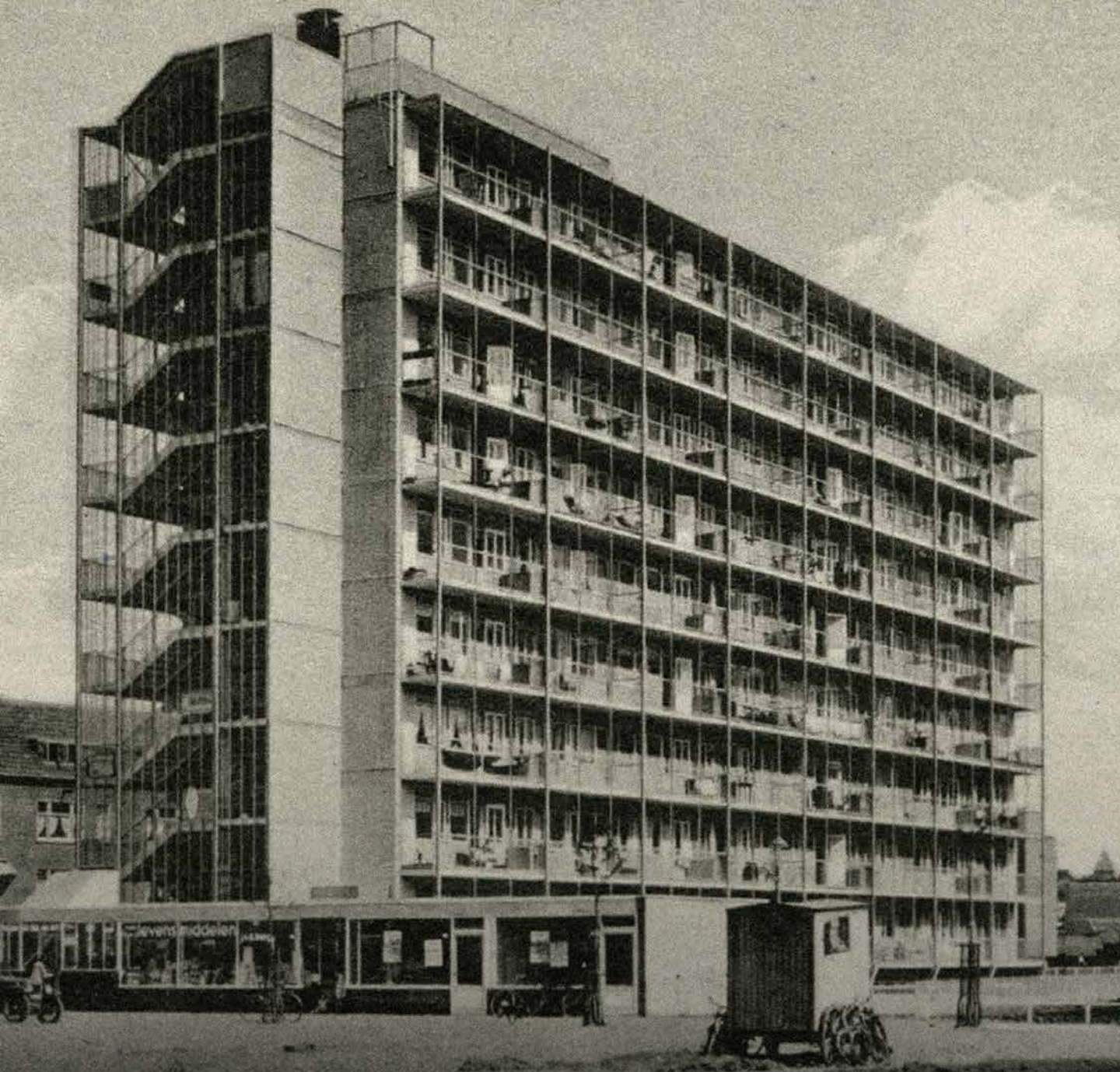
The Rotterdam Berpolderflat, designed by W van Tijen with Brinkman & Van der Vlucht, completed in 1934 (c.1934; SAR: NL-RtSA_4029_PBK-8057-01).
