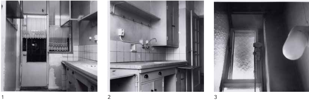
FIG. 6.19 The AWW Versteeg kitchen, photographed in Charlotte de Bourbon Street 34 in 1981. Note the [1] glazed extraction hood; [2] the pull-out counter; and [3] the pivot window and potlicht (H Veen; SAA: [1] 010122052677; [2] 010122052678; [3] 010122052679).
