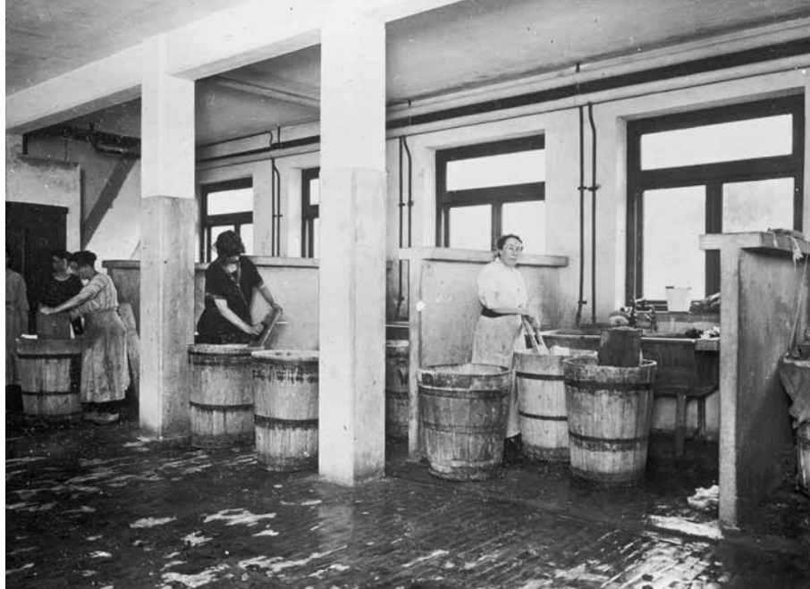
FIG. 5.15 A photograph of the laundry shortly after completion (J Frijhof; Housden, 1960, p. 158).
