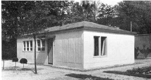
FIG. 7.7 The Acia house (Havenith, 1953a, p. 309).
