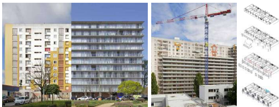
FIG. 5.5 Grand Parc Bordeaux, before and after the renovation project
