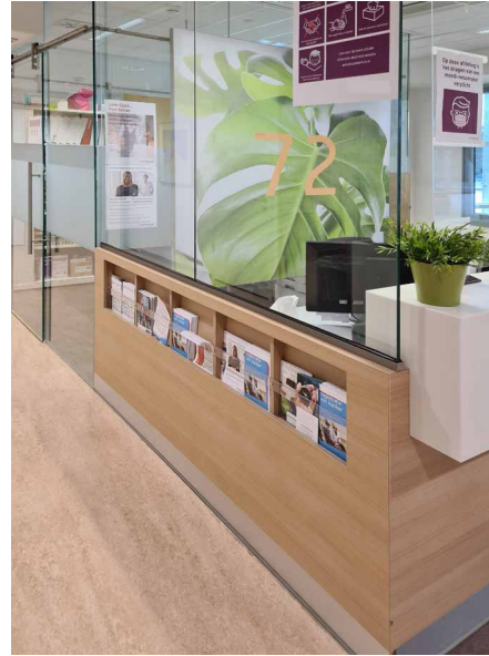
FIG. 6.7 Splash guard installed at reception. (photograph taken by a participant)
