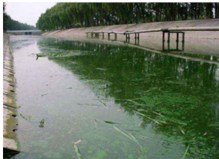
1 Inner-rivers are narrowed by concrete dykes
