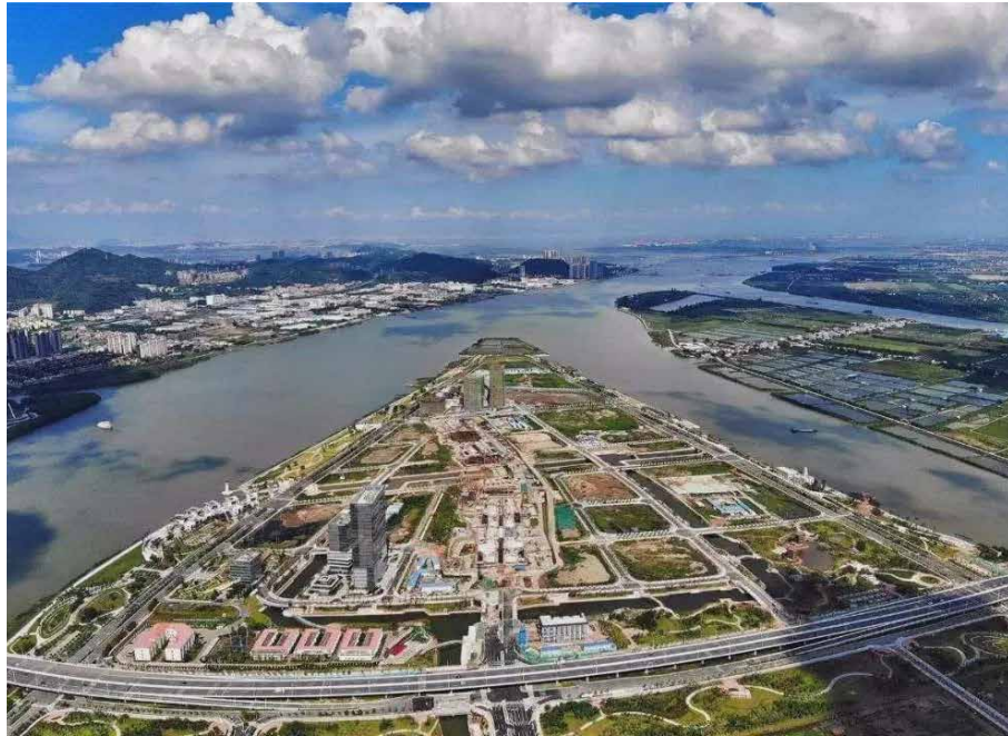
FIG. 5.9 Glimpse of Pearl Bay under construction
