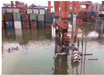
3 Tidal flooding causes malfunction of international port
