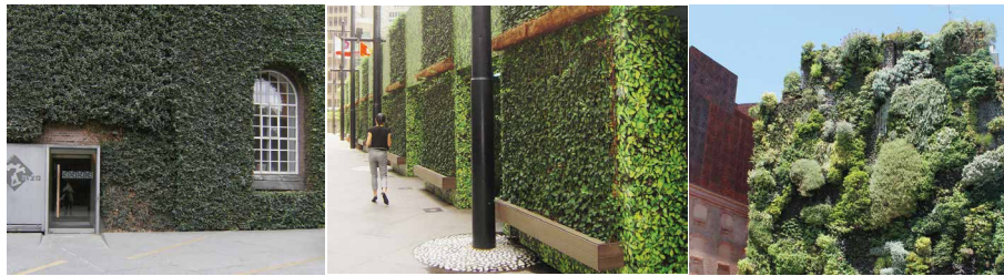
FIG. 8.2 From left to right: direct green façades, indirect green façades, living wall system
