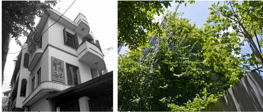
FIG. 8.1 A housing refurbishment case in Vietnam. Left: old house. Right: refurbished house
