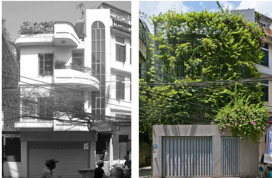
FIG. 3.1 Le Binh House before (left) and after (right) refurbishment
