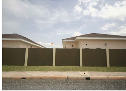
FIG. 7.6 Gated community in Appolonia Affordable housing options in Appolonia start at USD 70,000, which is far out of reach for most Ghanaians. Source: Author, 2019
