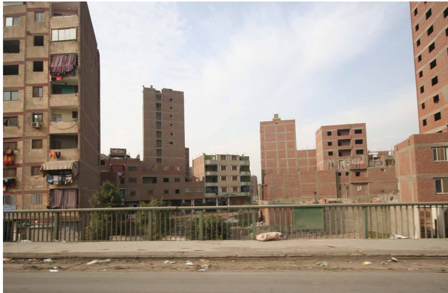
FIG. 5.6 Unregulated housing in Cairo
