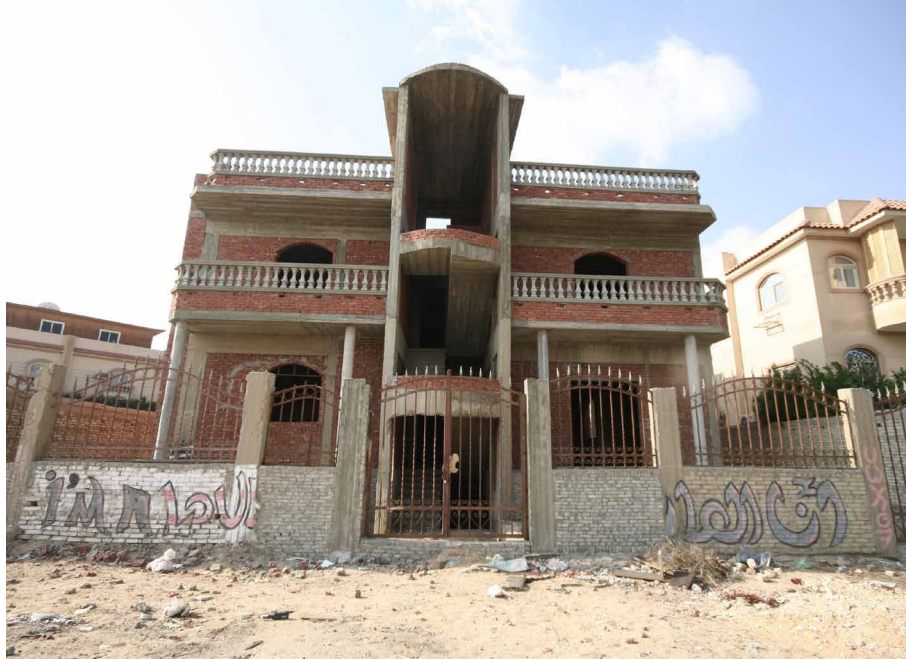
FIG. 5.5 Unfinished construction in Sheikh Zayed City, Egypt
