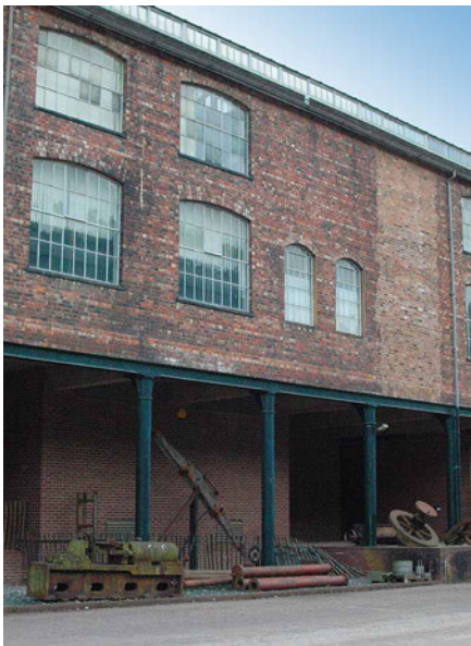
FIG. 1.20 Exterior of the converted Long warehouse after its conservation. The exterior intervention has respected the historic fabric, 2015.
