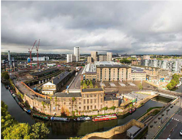
FIG. 5.7 View from the roof of Five Pancras Square, to the Fish and Coal Office, the Granary Square and the transformed Goods Yard. On the left, the image illustrates the Coal drops yard still underused and the re-erection of the first gasholder (John Sturrock).
