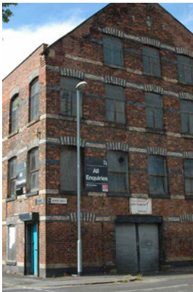
FIG. 4.16 Abandoned former industrial building located at the northeastern part of Ancoats. 2015.
