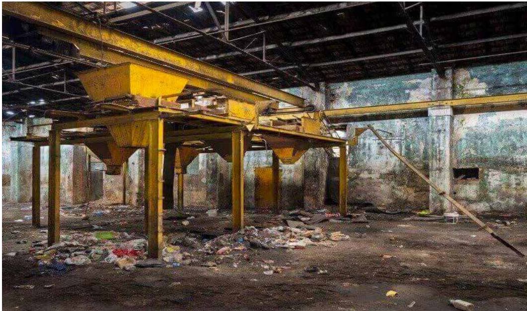
FIG. 15.4 Interior view of the former factory before its reuse, depicting machinery parts that were not preserved (Frank Gómez).
