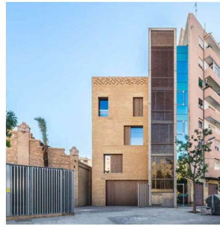
FIG. 15.14 The Day Centre for children and teenagers at risk of social exclusion (Ramon Esteve Architecture Design, n.d.).
