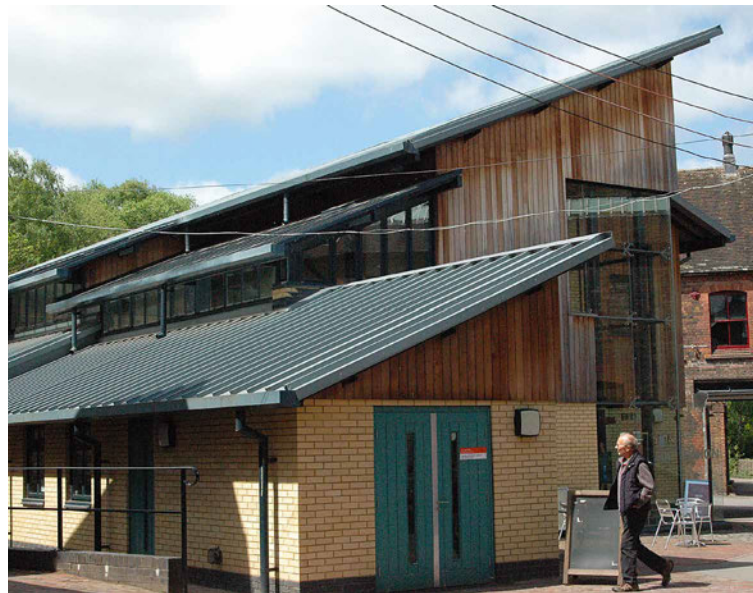
FIG. 1.21 Fusion, the new extension of the Jackfield Tile Museum presents little compatibility with the historic structures, 2015.
