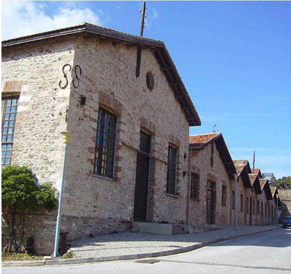
FIG. 18.6 The machinery building that will house the LMMM is one of the oldest and most renowned ones in Greece (Urban environment Laboratory, NTUA).
