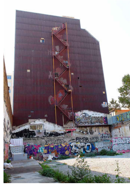
FIG. 13.6 Demolished industry in Poblenou, awaiting for development, 2017.
