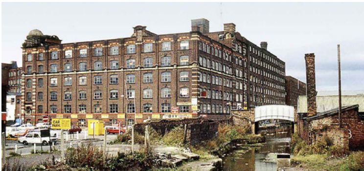
FIG. 4.5 The Royal Mills in decay in 1970 (heritagephotoarchive.co.uk).
