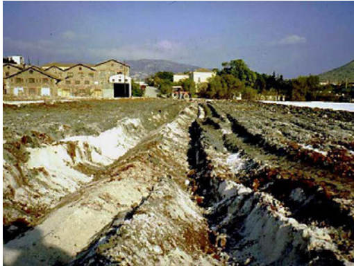
FIG. 18.3 Soil decontamination in the LCTP (Urban Environment Laboratory, NTUA).
