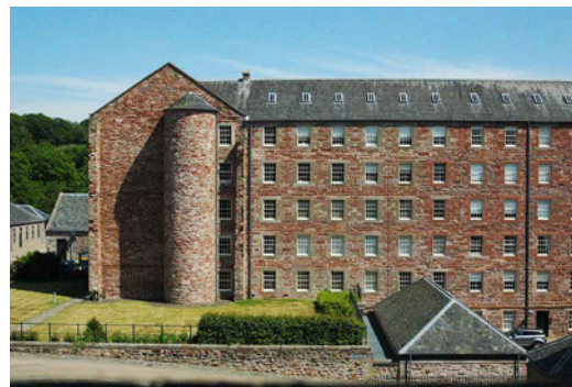
FIG. 3.6 The restored East Mill in 2015.
