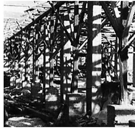
FIG. 19.4 The shed in 1998 after the addition of concrete columns (Kizis, 1999, 28).
