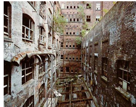
FIG. 4.6 Interior view of the Royal Mills in decay in 1980 (heritagephotoarchive.co.uk).
