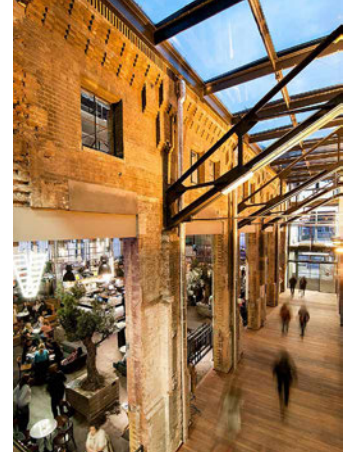
FIG. 10.11 The steel trusses and the rough brick wall are preserved, maintaining the industrial character of the building (Tim Leguijt Fotografie).
