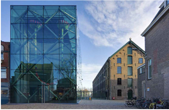
FIG. 7.10 The entrance building designed by cepezed (cepezed, n.d.).
