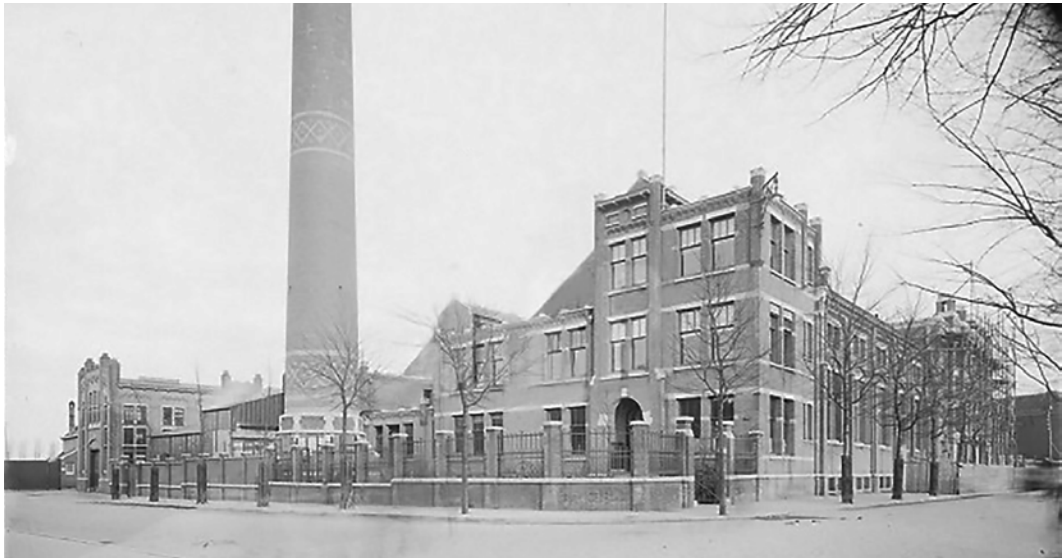
FIG. 10.2 The Energiehuis in 1910 during the construction of machine hall 2 and boiler hall 2 (Jonkman Klinkhamer architecten, 2009, 5).
