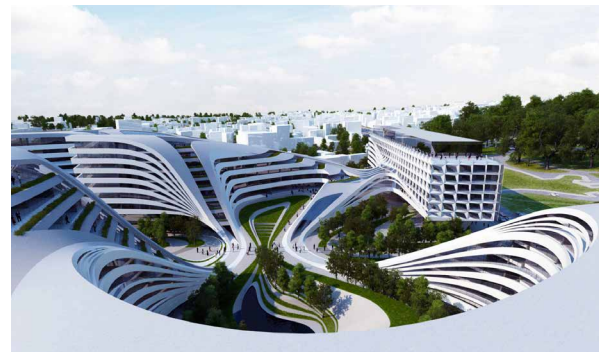
FIG. 6.6 The Bako masterplan in Belgrade by Zaha Hadid Architects involving the conversion of an old factory to a mixed use scheme. The character of the factory is largely overshadowed by signature architecture ( http://www.dezeen.com/2012/12/05/beko-masterplan-by-zaha-hadid/ ).
