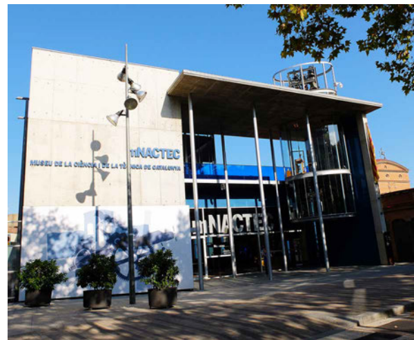
FIG. 11.5 Entrance building of mNACTEC, 2017.
