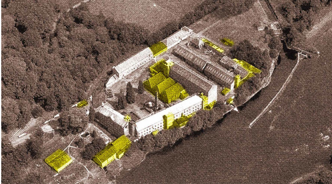
FIG. 3.2 Aerial photograph of Stanley Mills before demolitions. The building and features highlighted with yellow have been demolished (Cressey and Fitzgerald, 2011, 17).
