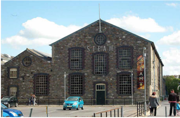
FIG. 2.3 The D Shop of GWRW converted into the STEAM Museum, 2015.
