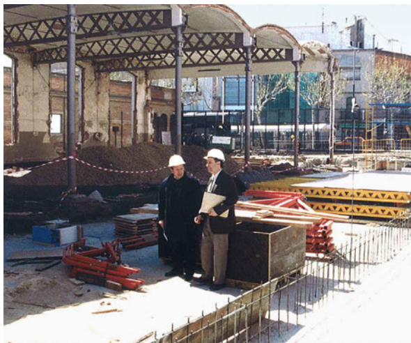
FIG. 11.4 Former warehouse during its transformation. (mNACTEC documentation centre).
