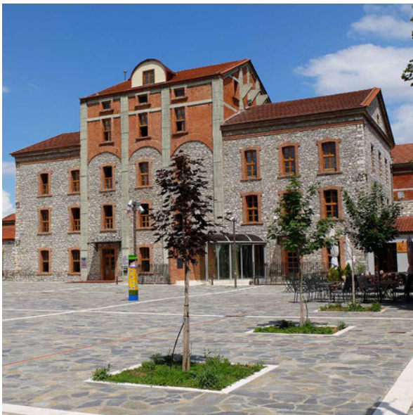
FIG. 20.11 The centrepiece of the Mill after its reuse, 2017.
