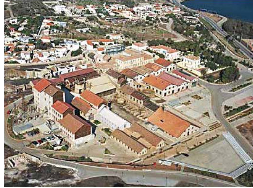
FIG. 18.4 The buildings of zone A after their restoration (Lavrion Technological and Cultural Park.).
