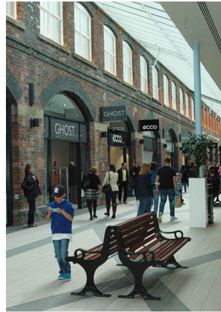
FIG. 2.15 The extension of the Designer Outlet to the foundry building, 2015.
