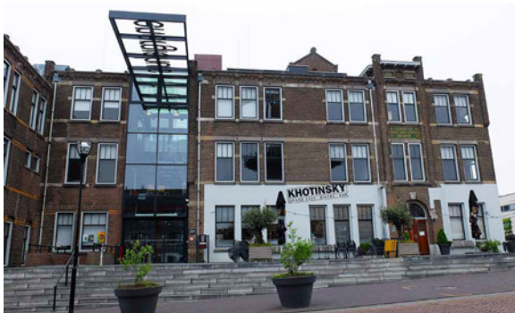
FIG. 10.7 The main entrance as part of the 'cut', 2016.
