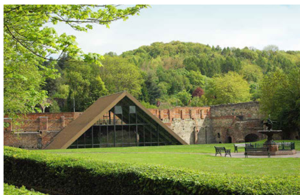
FIG. 1.17 The cover building of the Old furnace dominating the industrial ruins, 2015.
