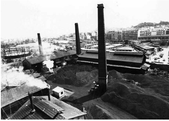
FIG. 17.3 The central courtyard of the gasworks before their conversion (Archive of preindustrial and industrial monuments, Directorate of Protection and Restoration of Modern and Contemporary Monuments).
