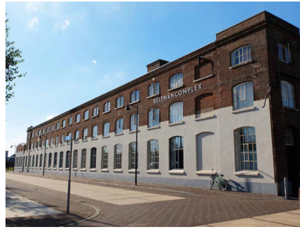
FIG. 9.3 The Beltman complex transformed into social housing, office space for rent and the offices of the Housing Corporation Woning, 2016.
