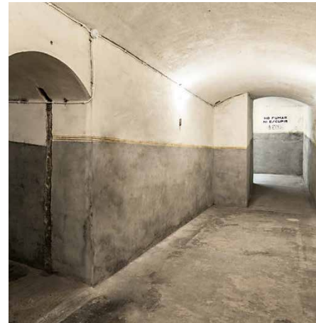
FIG. 15.12 The restored 20 th Cent. Civil War shelter (Bombas Gens Centre d'Art. n.d.).
