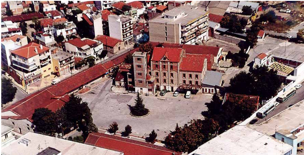
FIG. 20.4 The Mill of Pappas in 2001 (Municipality of Larissa - Directorate of Technical Services - Section of New Projects, 2011, 15).
