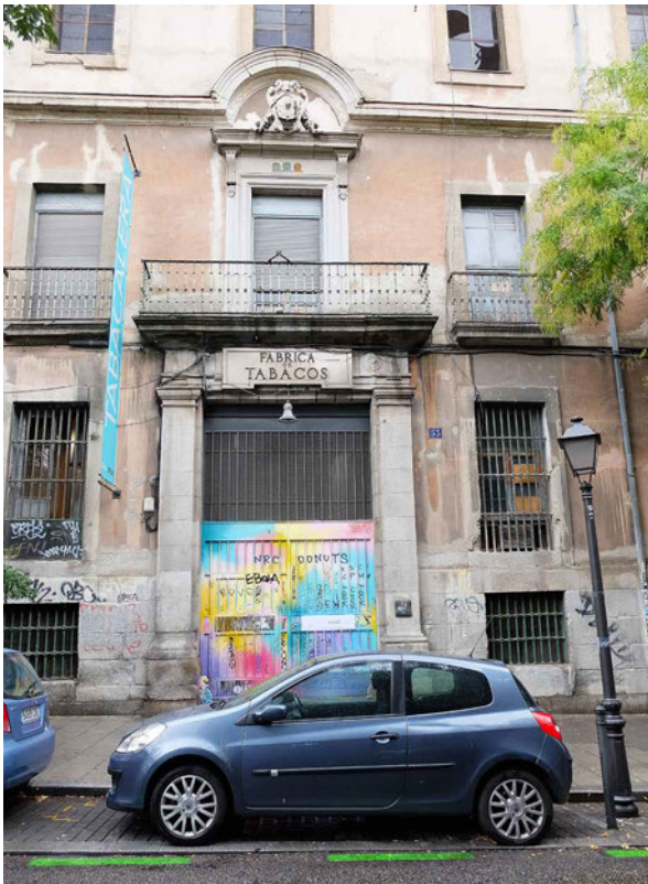
FIG. 14.7 The Tabacalera's main entrance, 2017.
