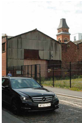
FIG. 4.17 Warehouses and empty lots behind the Cutting Room Square. 2015.
