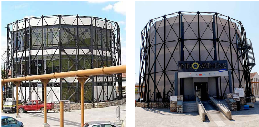
FIG. 17.7 The Gasholder of Technopolis before and after its latest renovation for housing INNOVATHENS (left photo: Ktizon blogspot, 2017).
