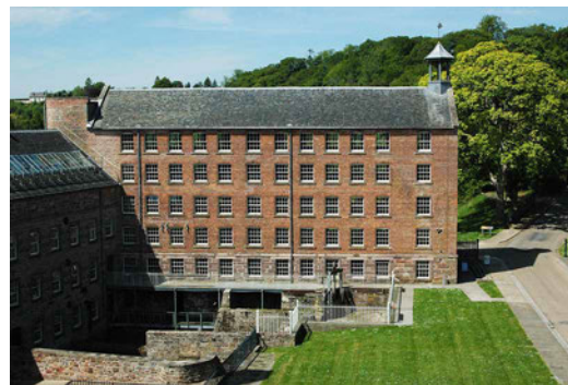
FIG. 3.4 The restored Bell mill and the excavated waterwheel pits in 2015.
