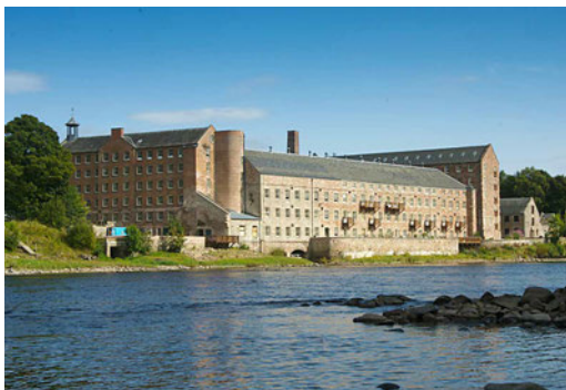
FIG. 3.5 The complex after its restoration from the opposite bank of Tay ( visitscotland.com ).
