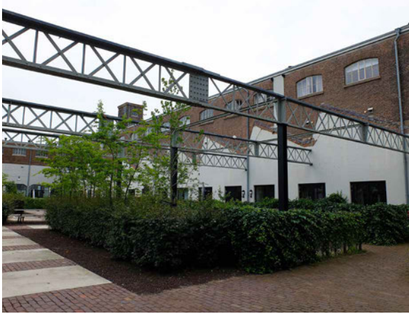
FIG. 9.2 The atrium of the Beltman complex. The roof of the industrial building has been removed for maximising the light in the residential and office units and allow for the creation of private and communal yards for the new users. The patina and structure of the historic building has been preserved, 2016.
