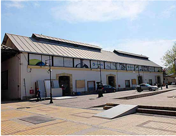
FIG. 17.5 The skylights of the new retort house serve as advertisement surfaces, 2017.
