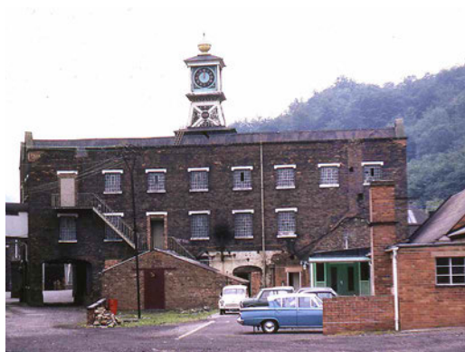
FIG. 1.9 The Great Warehouse in 1964 (IGM Archive).
