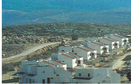
FIG. 4.56 Houses in Reut under construction, 1989. (IDF housing Administration)
