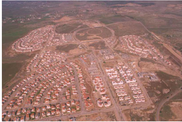
FIG. 5.17 First buildings in Shoham with the empty compounds in the north , 1995. Moshe Milner (GPO)
