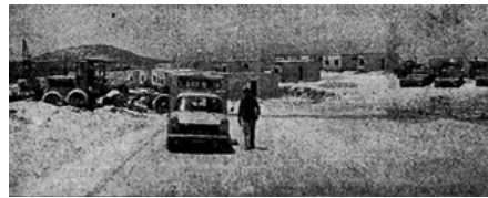
FIG. 3.24 Houses under construction in Hinanit, 1980. Amos Levav (Ma'ariv Newspaper)
