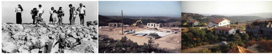
FIG. 3.3 A Joint tour to the site of the future settlement of Mitzpe Hila in the Upper Galilee, 1979; Construction of temporary houses in Mitzpe Hila; Permanent Houses in Mitzpe Hila, 1985. (Mitzpe Hila Council)
