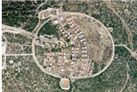
FIG. 3.26 Hinanit, 2005. (govmap.gov.il). Note the alterations to the old housing units in the eastern part, and the newly constructed ones in the western part
